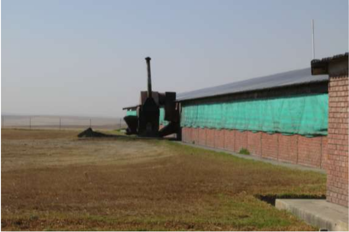
Figure 7: Photograph of a coal fired heater at the existing facility (1).
