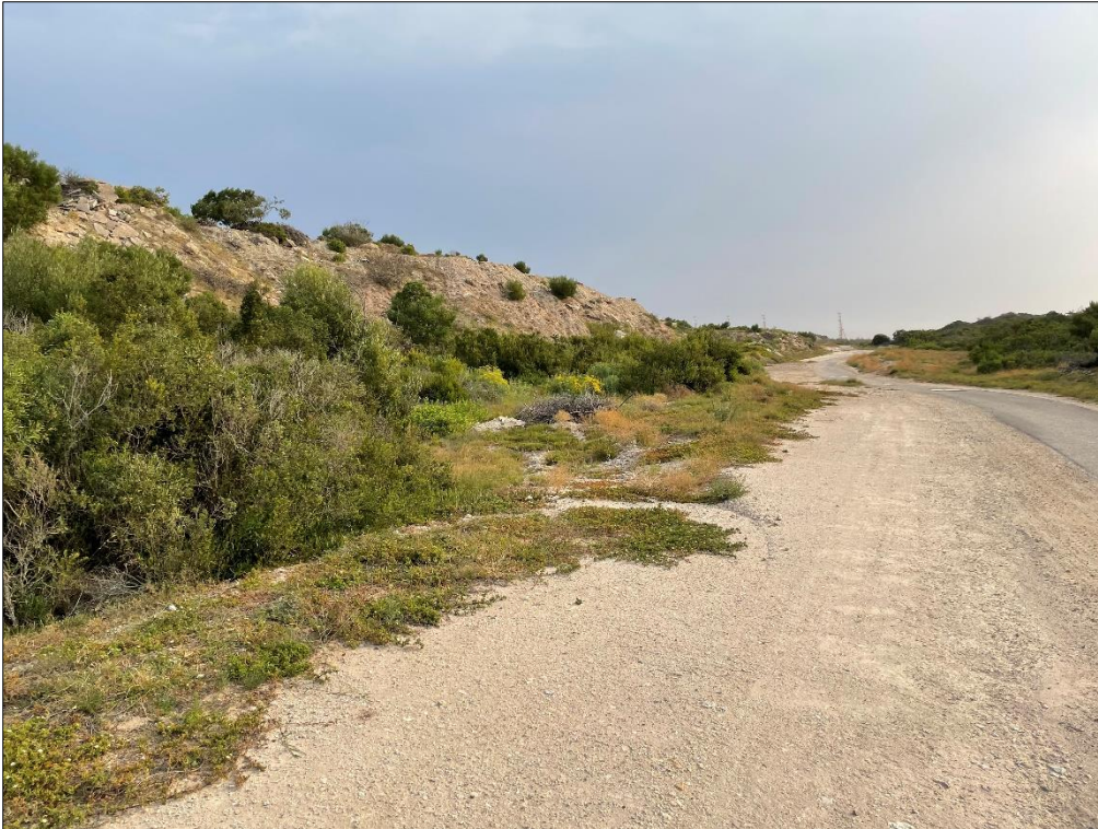
Figure 22. Zone 8. A short section of the transmission line will be aligned alongside the National Port Authority Road. Note the large berm alongside the road
