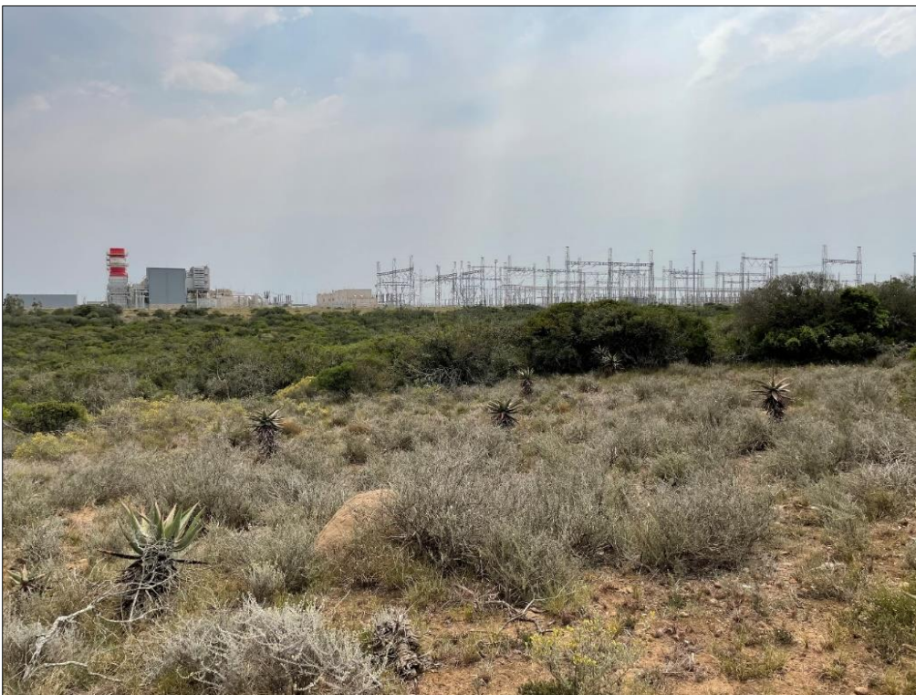
Figure 15. Zone 14 View of the preferred powerline servitude facing north. The Eskom Dedisa substation is in the background of the plate
