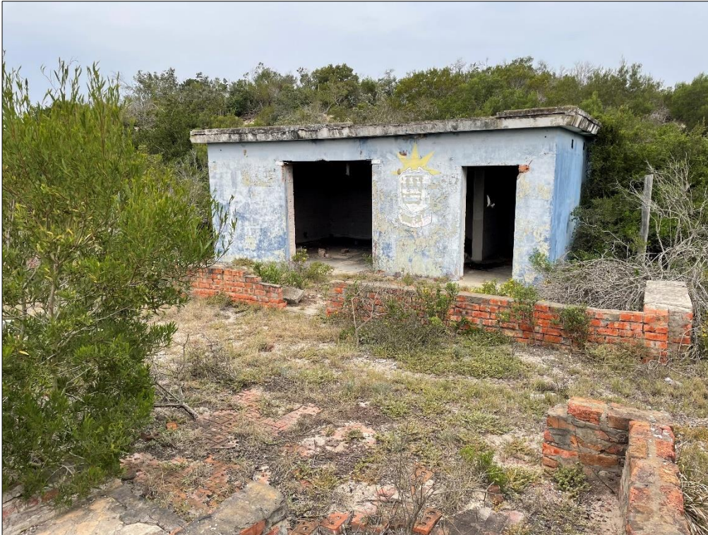
Figure 37. WWII Special Signal Services (SSS) Barracks (Sonop House)
