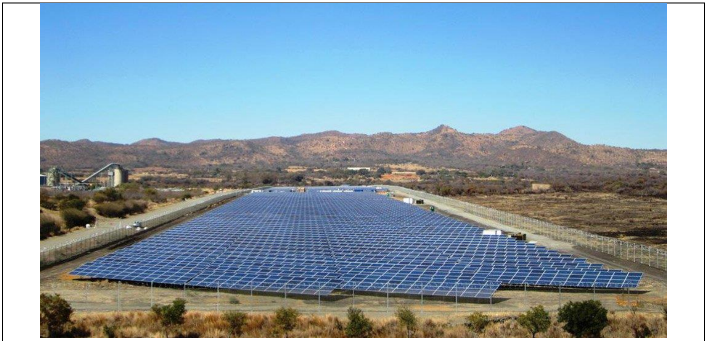
Figure 2.5 Photographs of the construction phase of a solar facility similar to the AMSA Vanderbijlpark Solar 3
