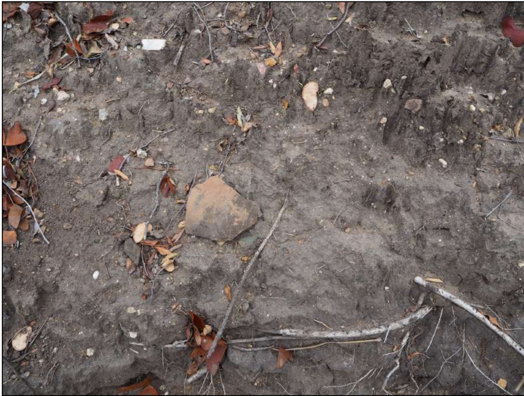
Figure 22. Deposits within vertical erosion wall
