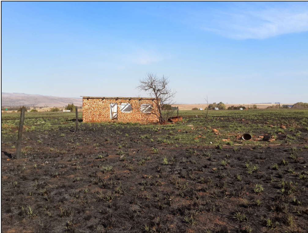
Figure 11: Recent structure on the study area viewed from the north (Lyd 1)
