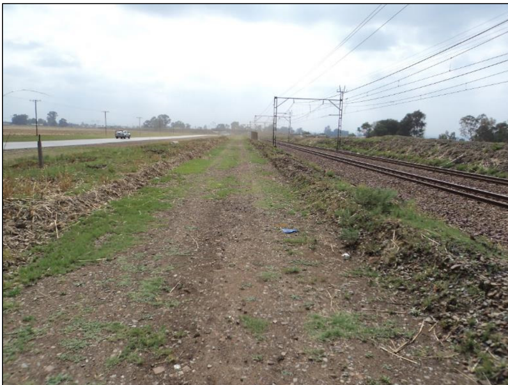
Figure 4: Environment from the western most point along the railway tracks.
