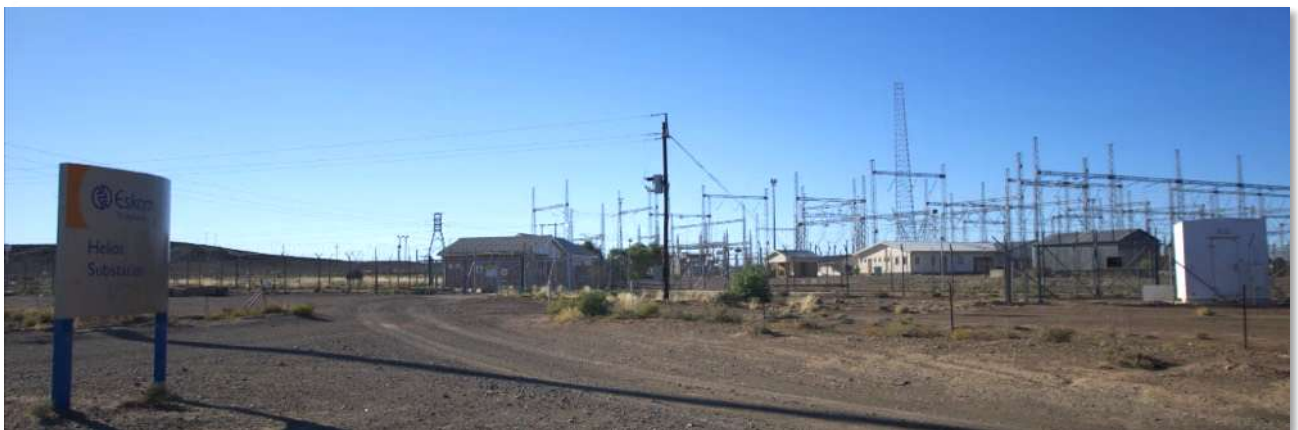
Figure 4-5: The Helios MTS east of the proposed Kokerboom WEF developments
