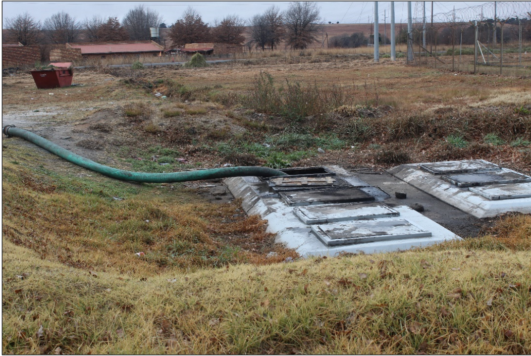
Figure 2: Existing underground septic tanks to be decommissioned.
