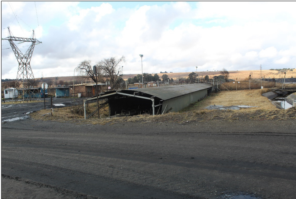
Figure 8: An old disused conveyor belt covered by a barrel roof.
