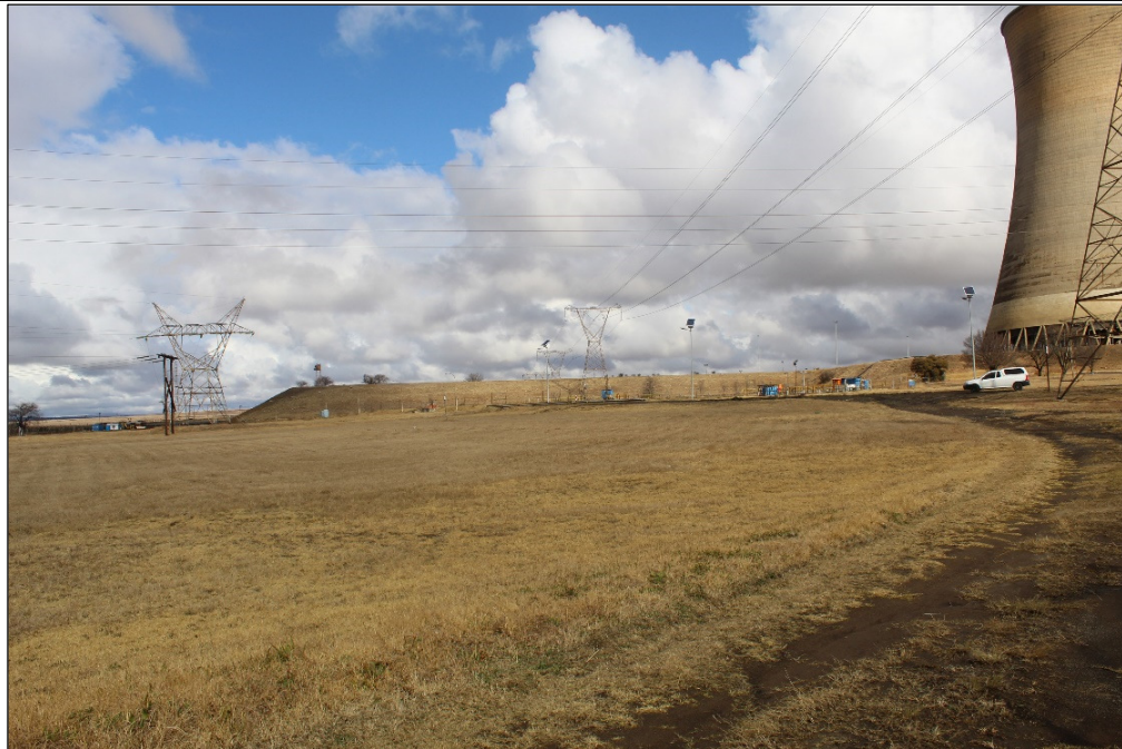
Figure 3: Site of installation of sewer pump in the foreground. Surface piping will be laid in the direction of the left end of the artificial terrace in the background.
