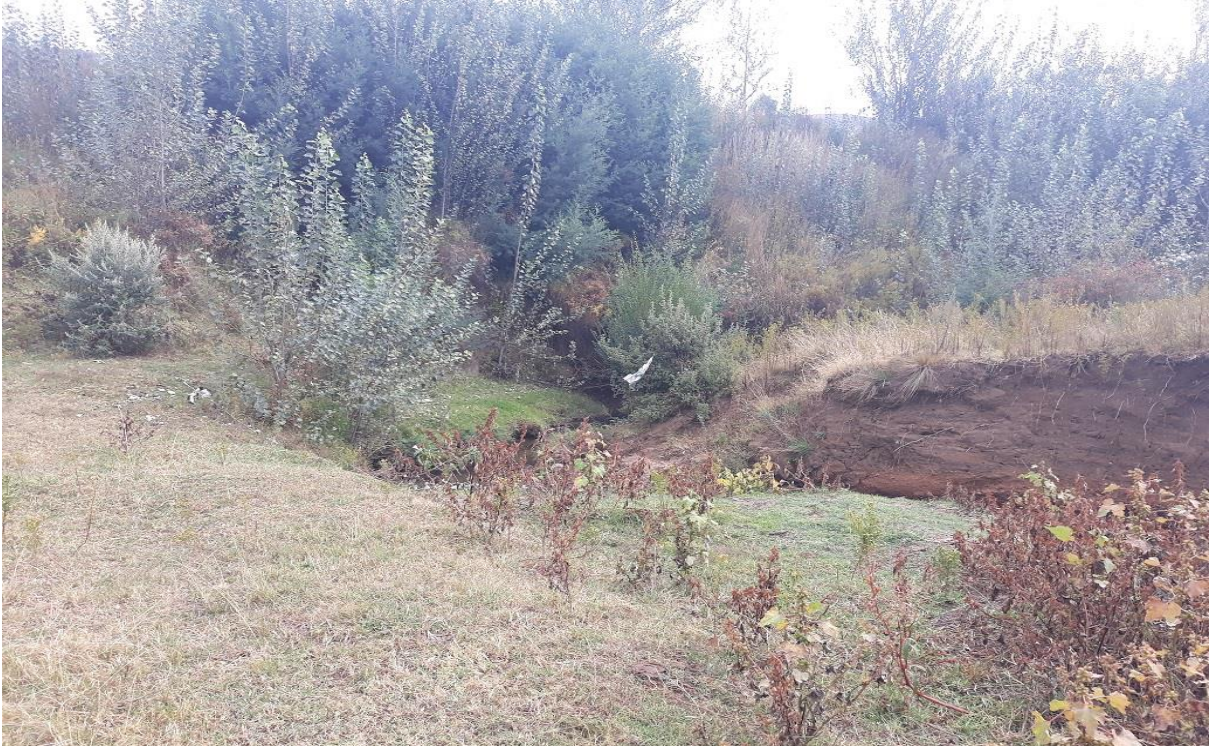
FIGURE 18: EMBANKMENTS AND VEGETATION GROWTH AT THE SELAHLIWE VILLAGE BRIDGE SITE.
