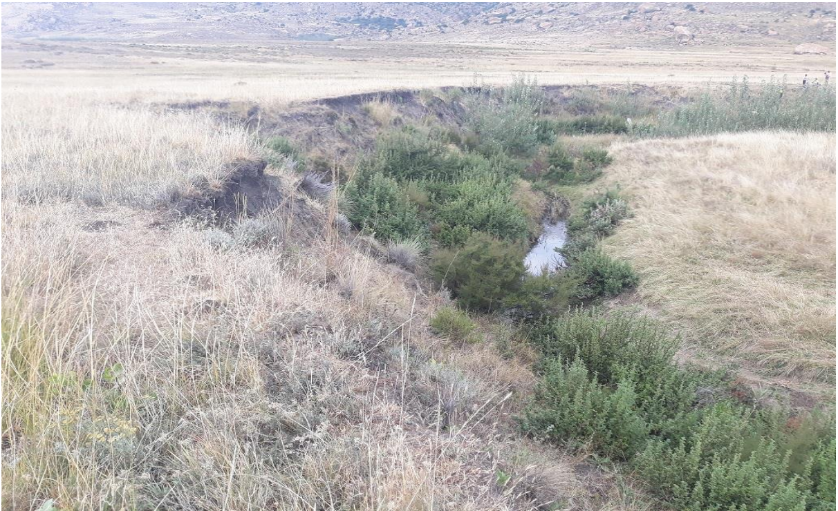
FIGURE 15: EMBANKMENTS AND VEGETATION GROWTH AT THE KHOSHENG VILLAGE BRIDGE SITE.
