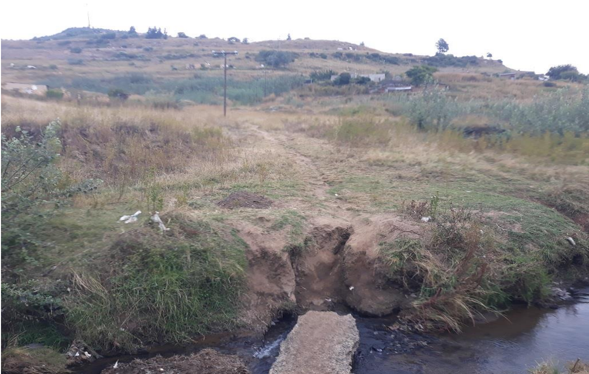
FIGURE 19: VIEW OF PROPOSED BRIDGE AREA FOR PHOPHOPHO VILLAGE.
