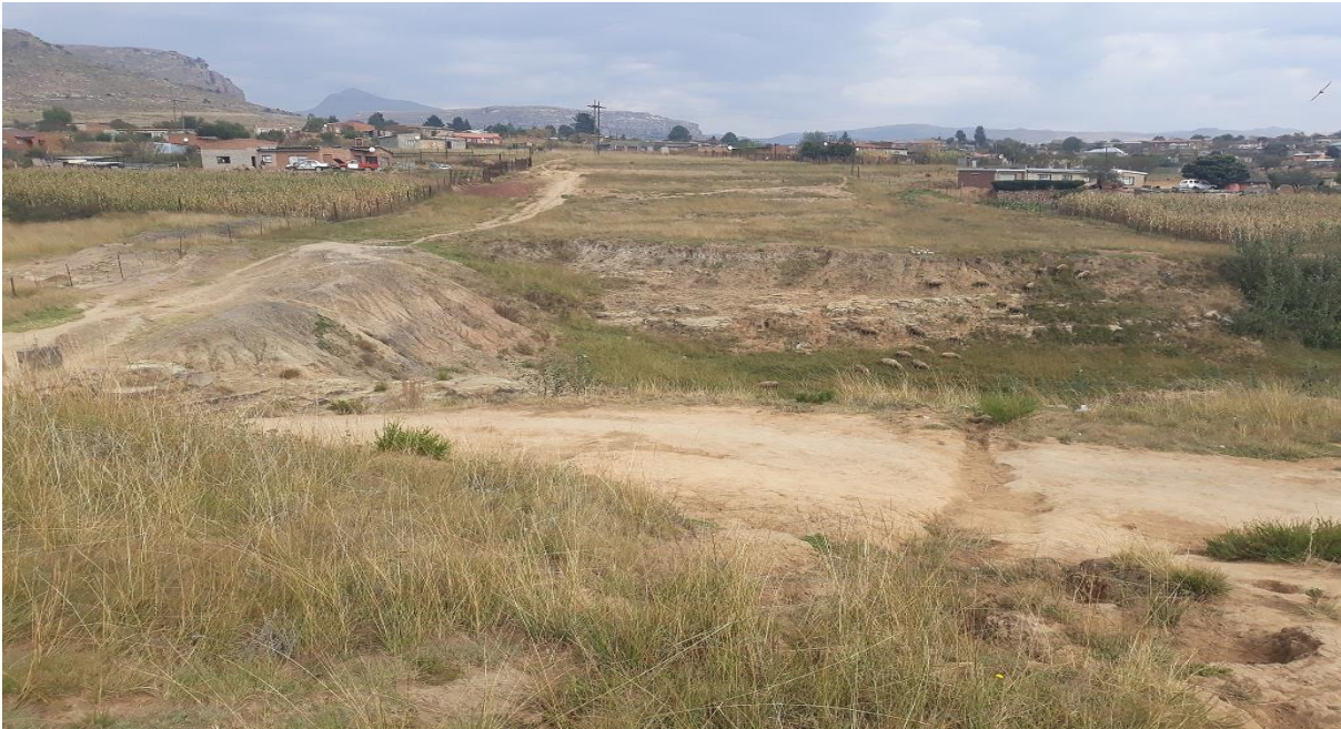
FIGURE 12: EMBANKMENTS AND VEGETATION GROWTH AT THE POELONG VILLAGE BRIDGE SITE.
