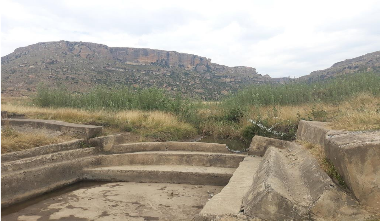
FIGURE 14: SMALL WATER CONTROL DAM AT THE KHOSHENG VILLAGE BRIDGE SITE.
