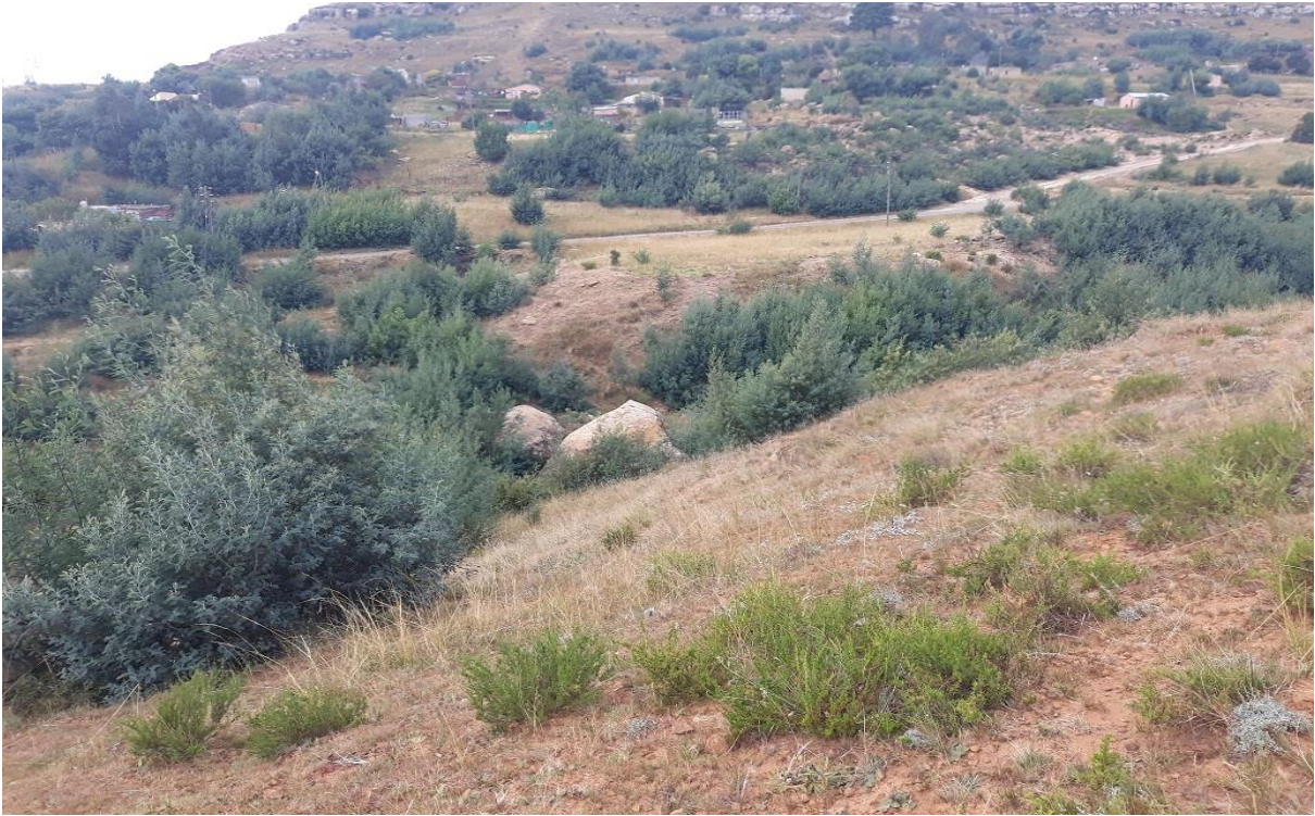
FIGURE 23: EMBANKMENTS AND VEGETATION GROWTH AT THE SEHLAJANENG VILLAGE BRIDGE SITE.
