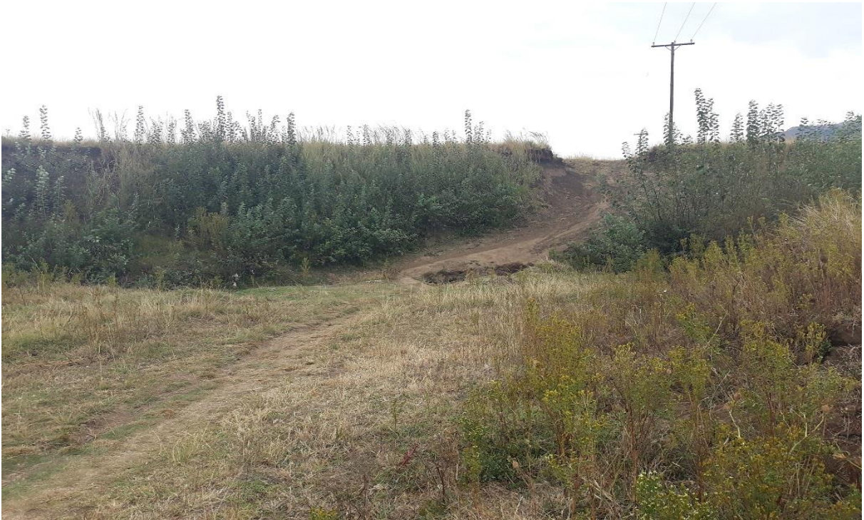
FIGURE 21: EMBANKMENTS AND VEGETATION GROWTH AT THE PHOPHOPHO VILLAGE BRIDGE SITE.
