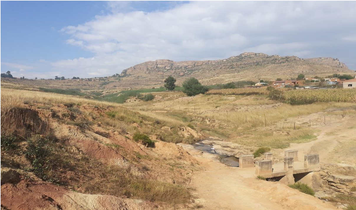
FIGURE 11: OLD FOOTBRIDGE AT THE POELONG VILLAGE BRIDGE SITE.
