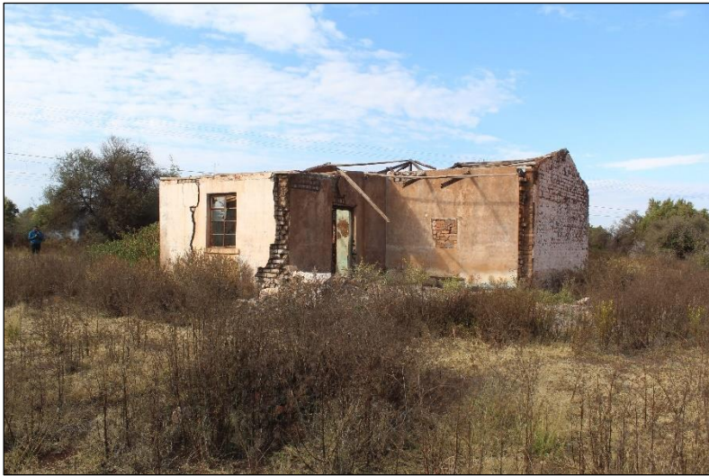
Figure 2: View of the east and north elevation of the building shows a room with two walls which have collapsed
