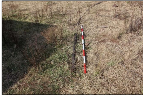
Figure 14: Polythene pipe for transportation of water
