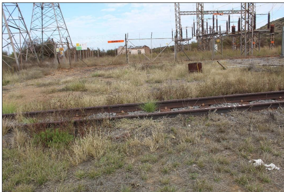
Figure 11: The old building, view west from a position behind the electrical substation
