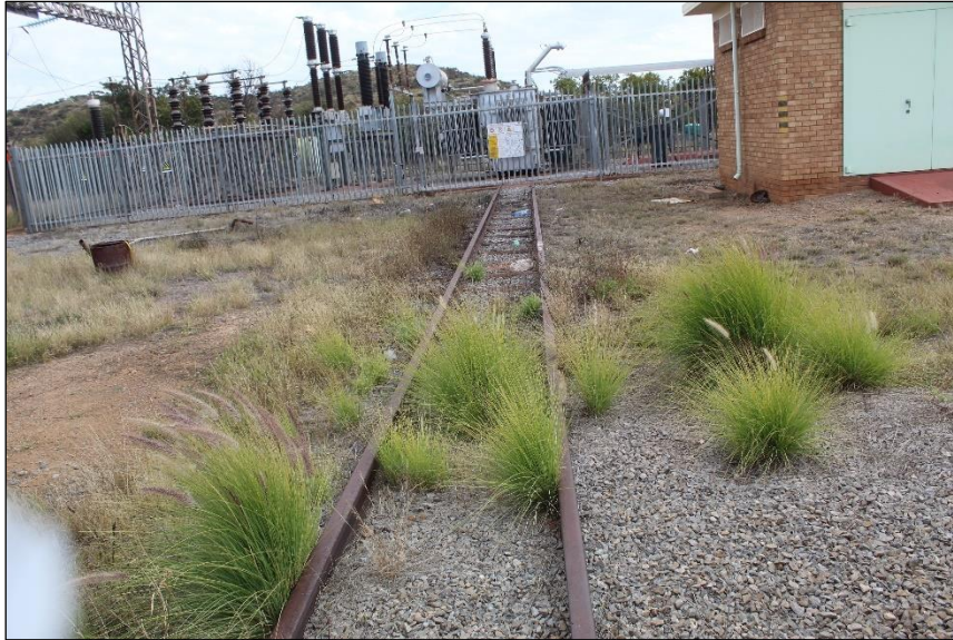
Figure 10: The electrical substation seen from the east. It was built at the terminal of a short railway line. The main line is behind the camera running parallel with the perimeter fencing of the substation in front of the camera.
