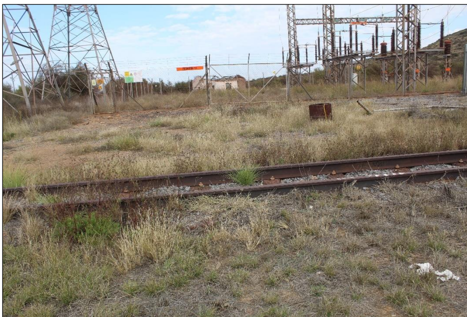
Figure 11: The old building, view west from a position behind the electrical substation
