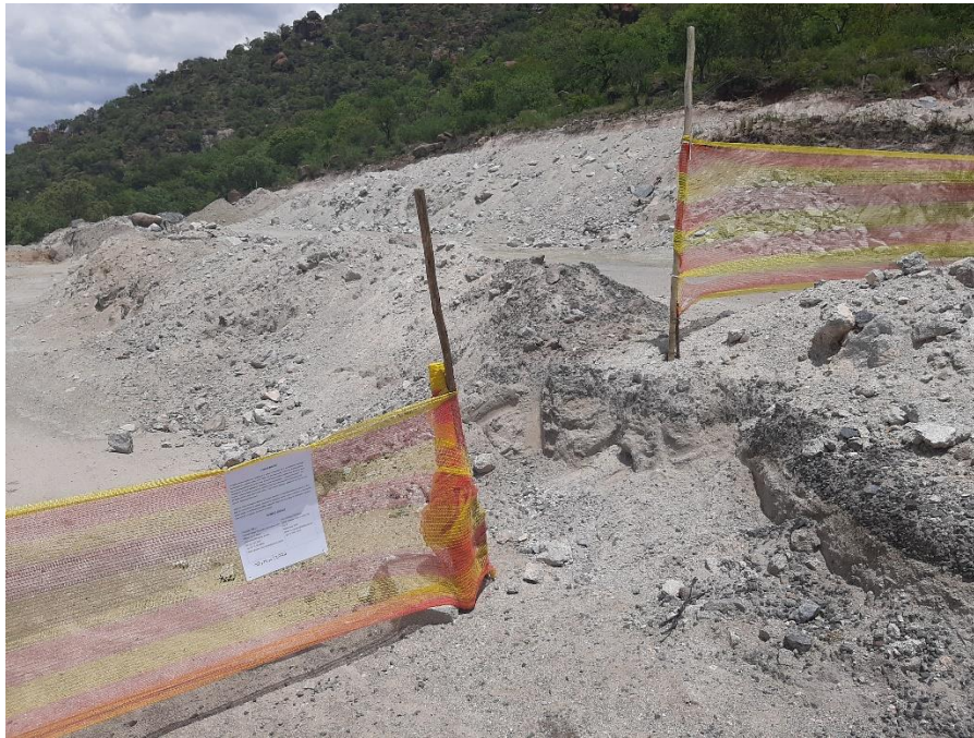
Figure 8: Public notice placed at the site of the earthworks
