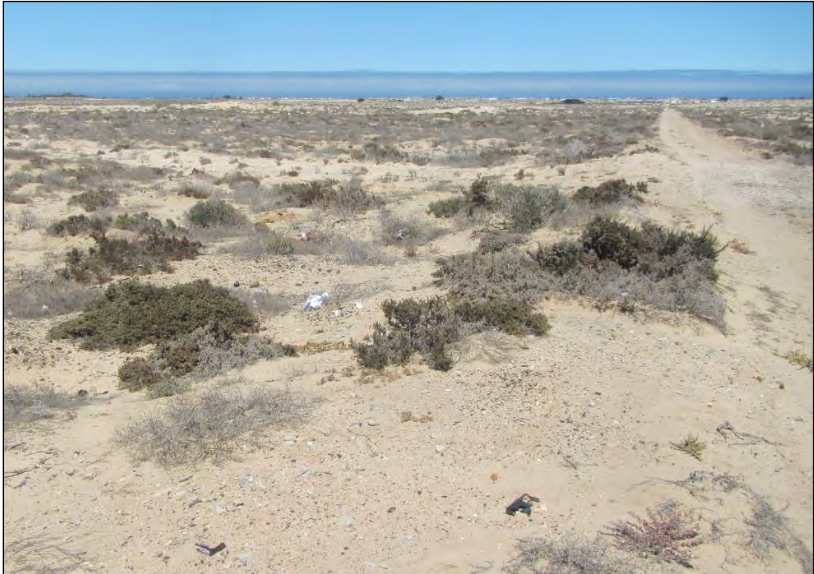
Figure 28: Looking towards the west along the railway berm (visible at right) and showing dumped materials (dark spots in the foreground) and the alignment of the trench that was unfortunately dug through the berm when the new oxidation ponds were built.
