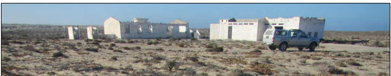
Figure 45: View of the old mine structures in Block S19.
