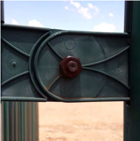
Fig 3 : weak connector between fence
