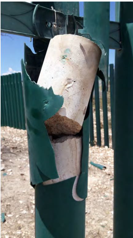
Fig 3 : weak connector between fence
