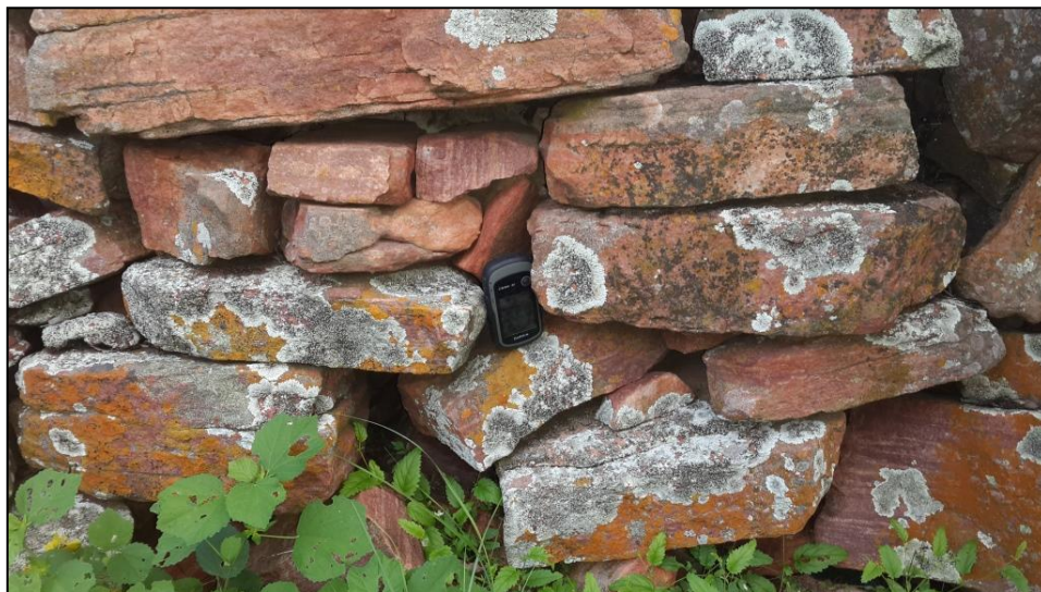
Figure 28: Late Iron Age walling on the farm Ketting (courtesy of Geoactive Dynamic Geological Services).
