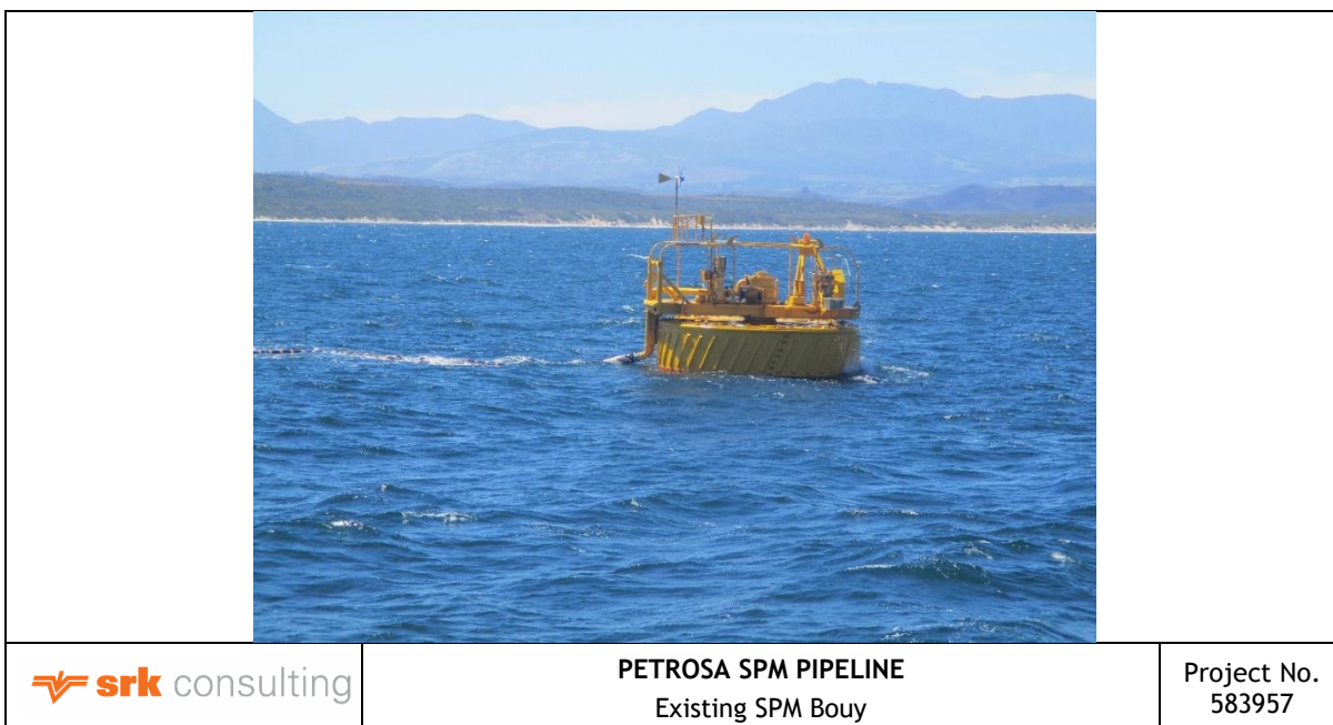
Figure 3-1: Existing SPM buoy
