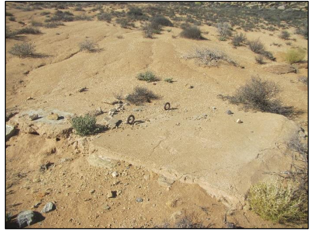
Figure 24: Iron loops in a cement foundation at Carolusberg.
