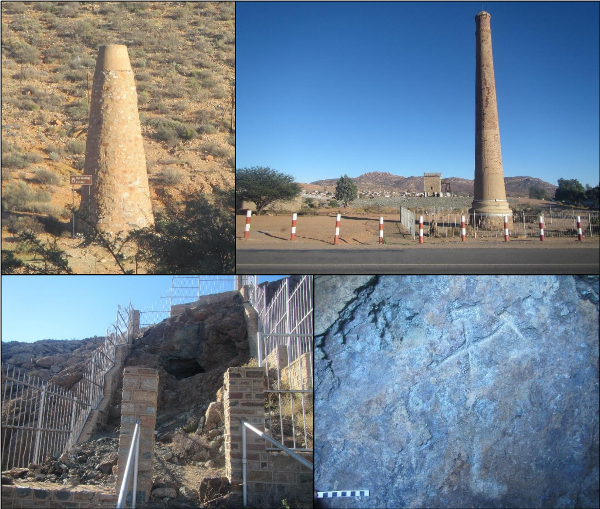
Figure 32: Provincial heritage sites related to copper mining in the region. Top left: smelting furnace at Springbok. Top right: Smoke stack with Cornish Beam Pump in the background at Okiep. Bottom: Simon van der Stel mine with mining symbol (scale in cm).
