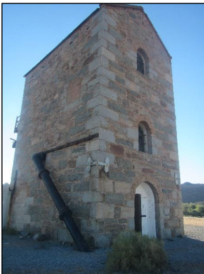
Figure 44: View of the southwest corner of the Cornish Beam Pump.
