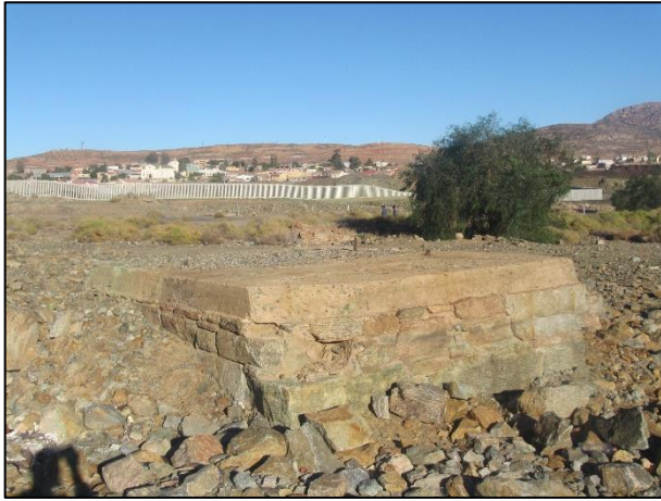
Figure 47: A stone foundation with concrete slab on top (waypoint 1896).
