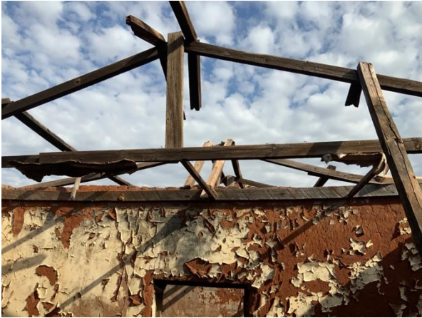
Figure 9. Detail of the truss structure and weathering internal wall paint
