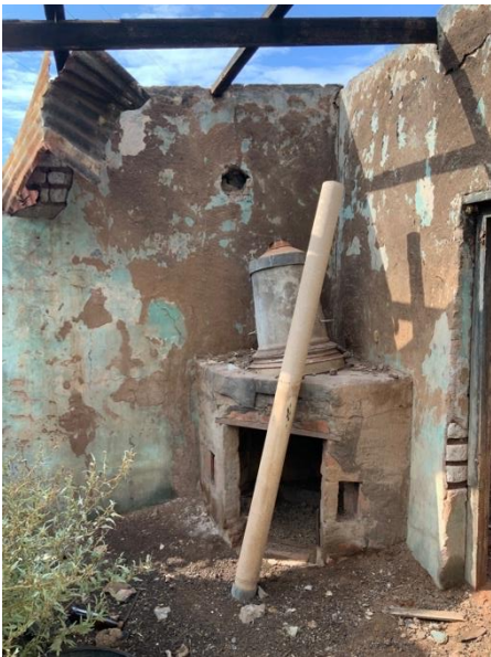
Figure 7. Detail of the kitchen
