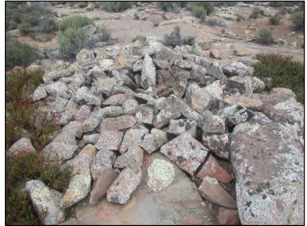
Figure 31: Collapsed circular stone-walled structure at waypoint 808 in Northern Cape (Sutherland WEF).
