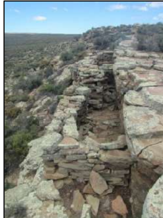
Figure 33: View towards the southwest of the structure at waypoint 806 with the cliff to the right.
