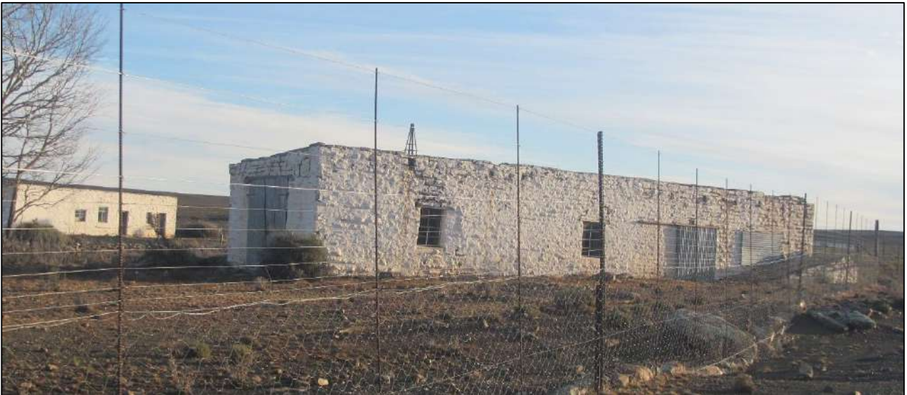
Figure 59: A stone-walled outbuilding in the Ou Plaas farm complex at waypoint 1165.
