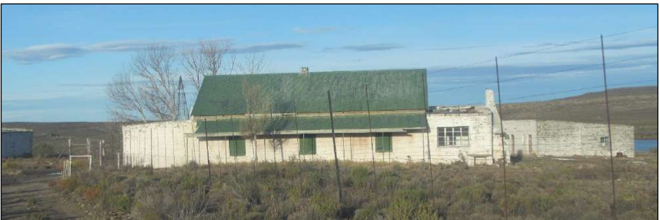
Figure 57: Western side of the abandoned farmhouse in the Ou Plaas farm complex at waypoint 1165. A veranda shades the three west-facing windows.
