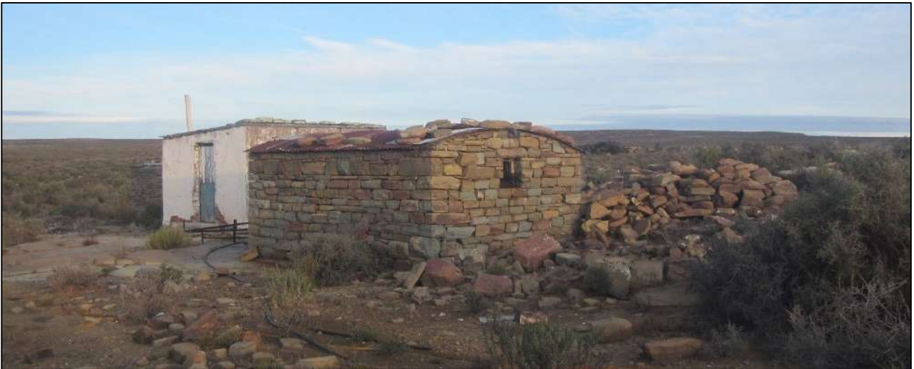
Figure 65: Stone structure within the Beerfontein farmstead at waypoint 1171a.
