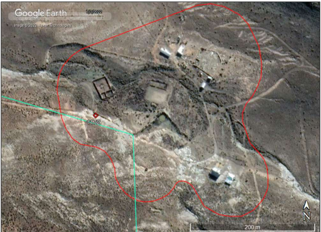
Figure 75: The powerline route (turquoise line) through the Beerfontein farm complex at waypoint 1172.
