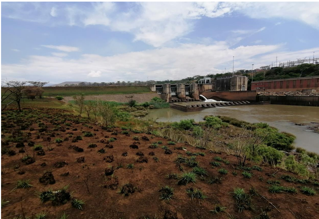
Photo Plate 6: A view of the Dam wall
