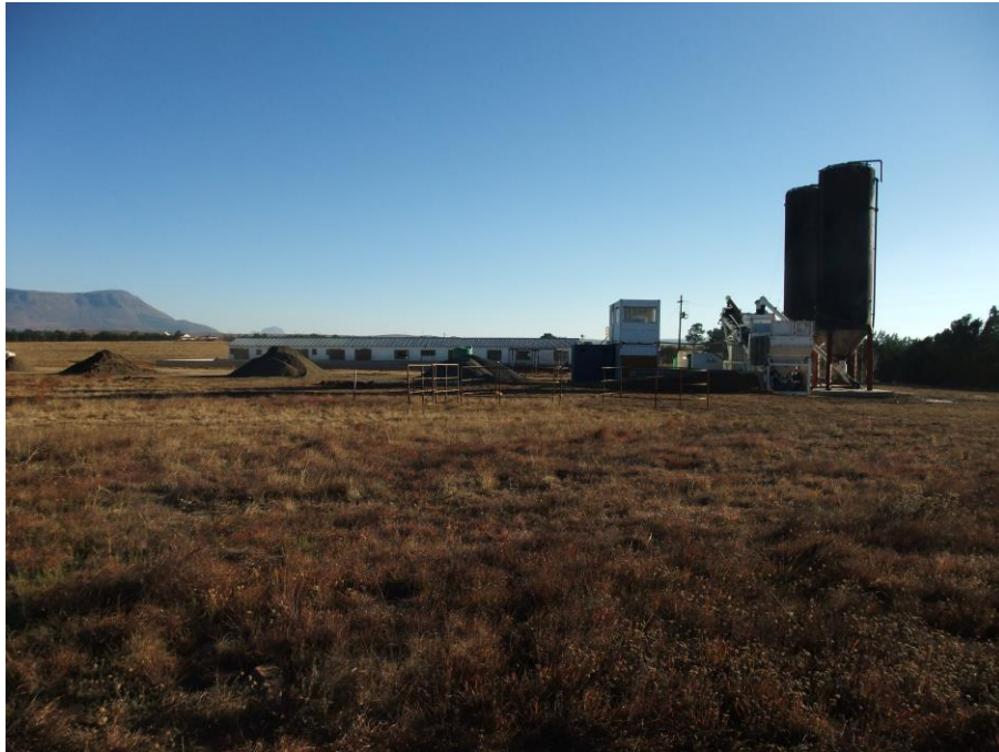
Figure 10: Building and other infrastructure on site.
