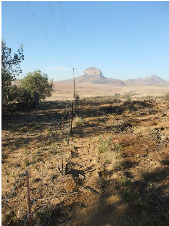
Figure 7: Disturbed area along the pipeline route.
