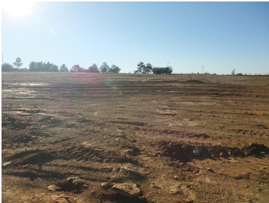
Figure 9: Earthwork activities on site.
