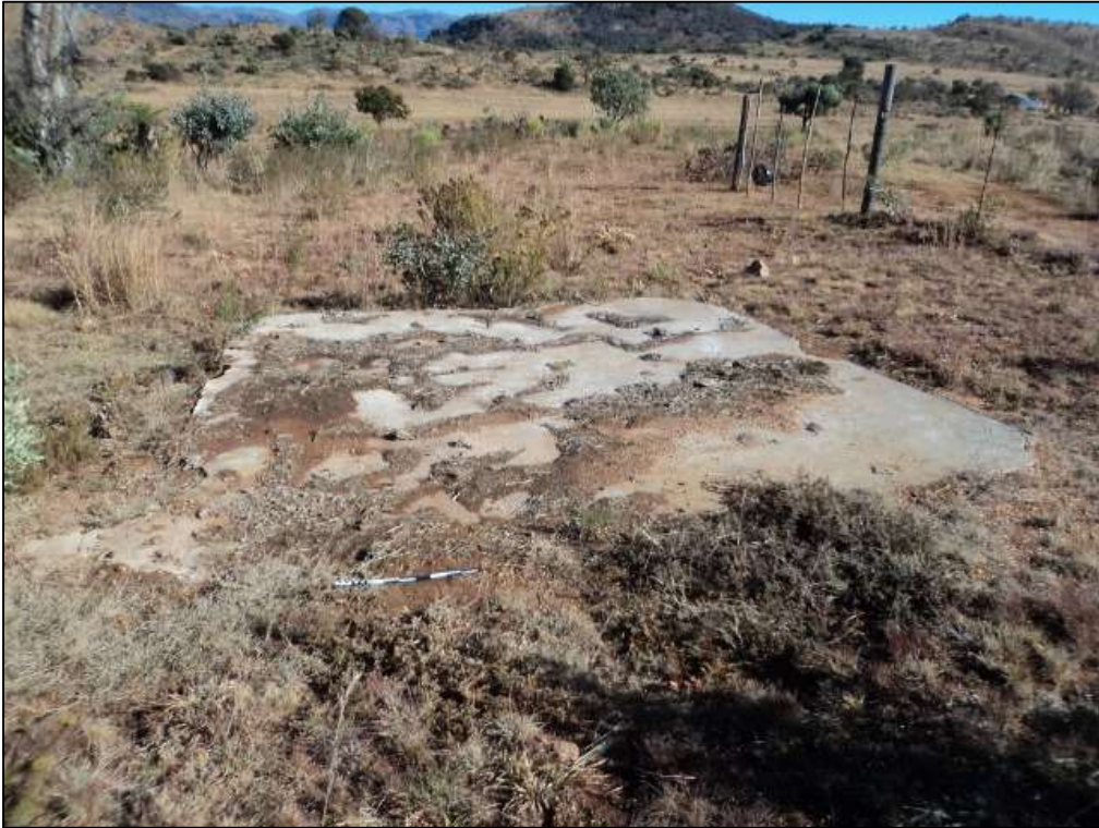
Figure 47: Modern foundation H01.
