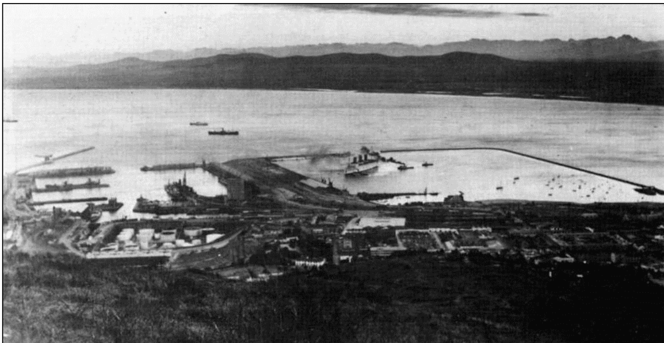
Plate 12: The new southern basin in 1934 with the random block mole at right (in Newall 1993)
