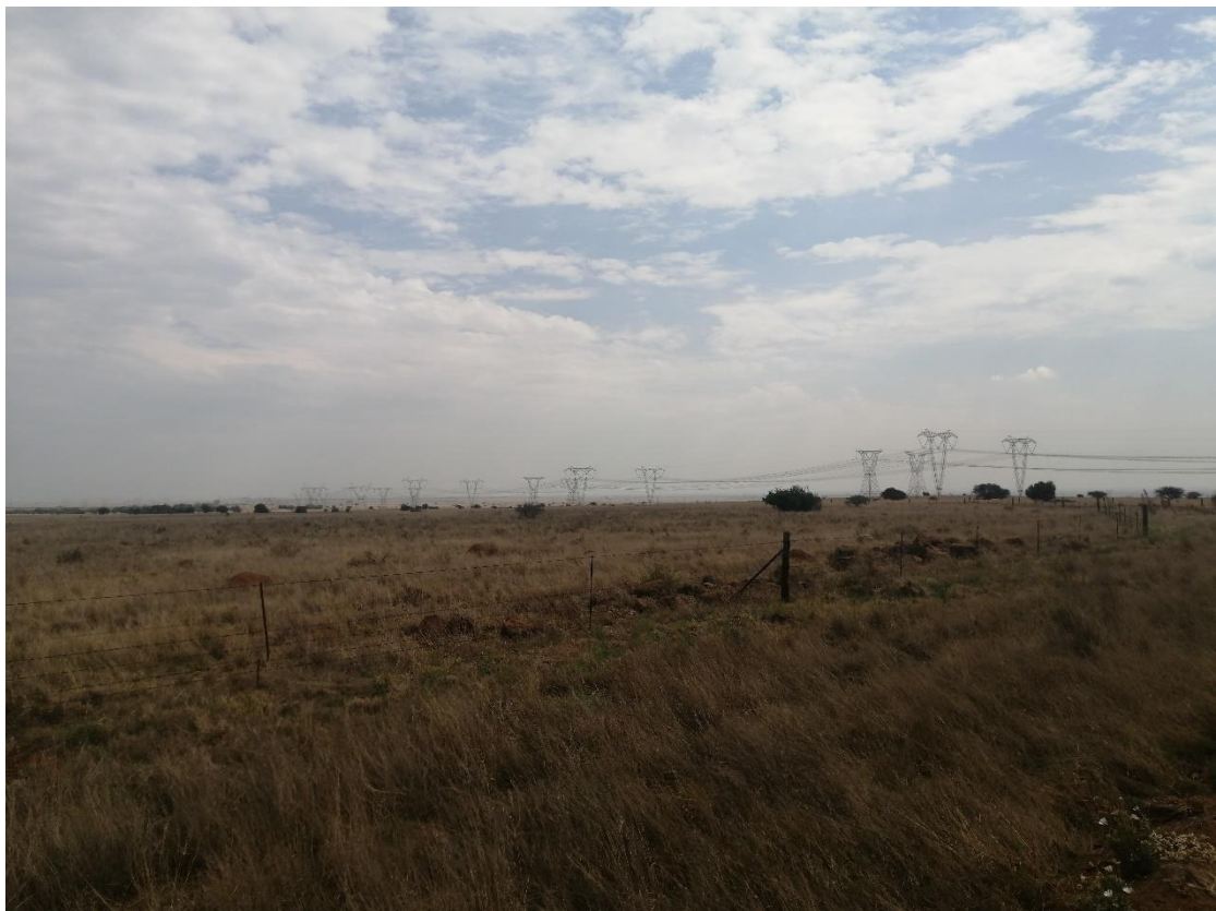
Figure 12: Example of the numerous power lines that traverse the area
