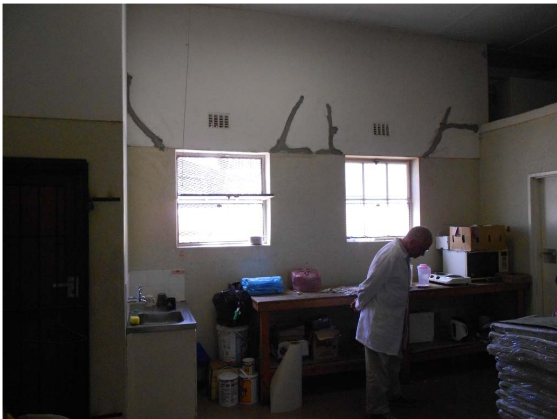
Photo 18: Inside the first floor of Atlas trading concrete framed building.
