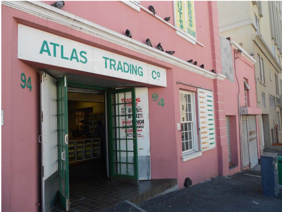
Photo 17: Entrance of Atlas Trading. Concrete frame structure constructed approximately 35 years ago.
