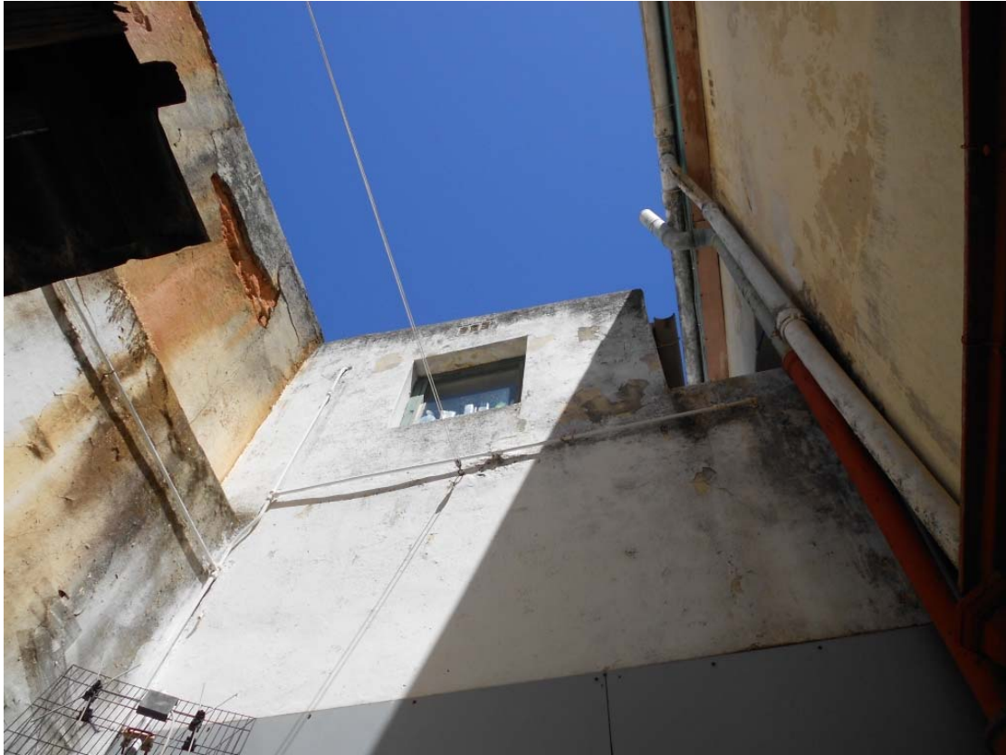
Photo 13: View inside back yard of barber shop. Note new independent wall adjacent stone wall.
