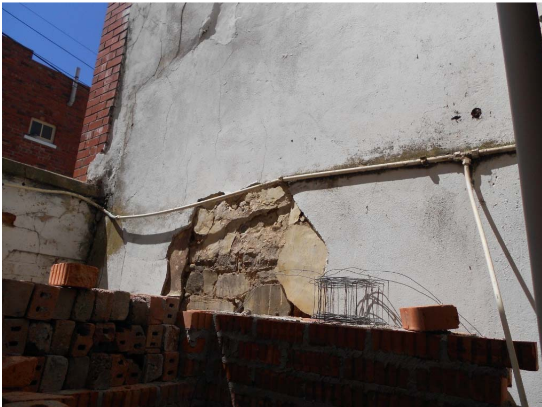
Photo 8: View inside Mohidien courtyard of new brickwork as well as existing plastered stone wall.
