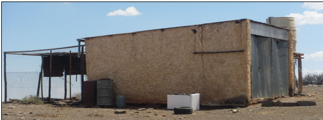
Figure 25: The farm outbuilding at waypoint 695 in the north-western corner of the study area.
