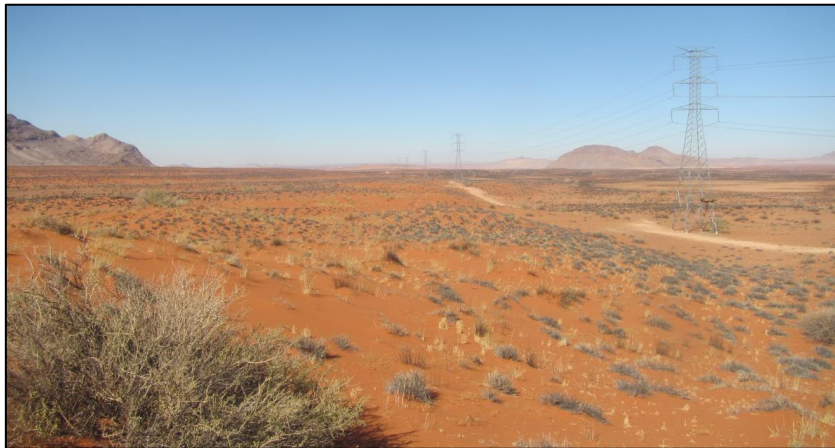
Figure 14: View towards the southeast across the dune area in the central part of the powerline route.
