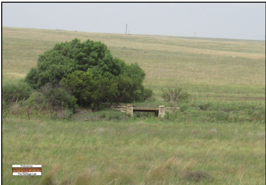
Figure 9. Ashlar built culvert on the original 1892 railway line
