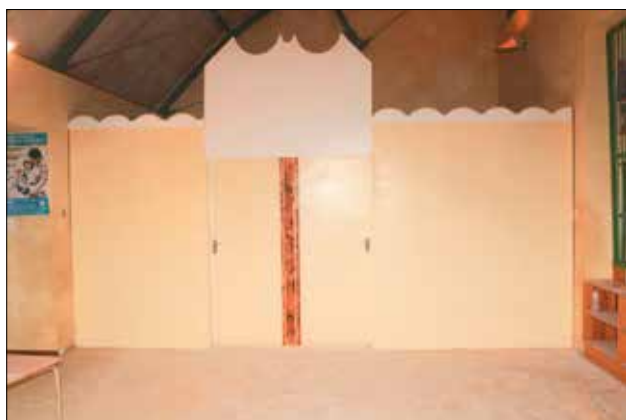
A view of the office after partitioning..
