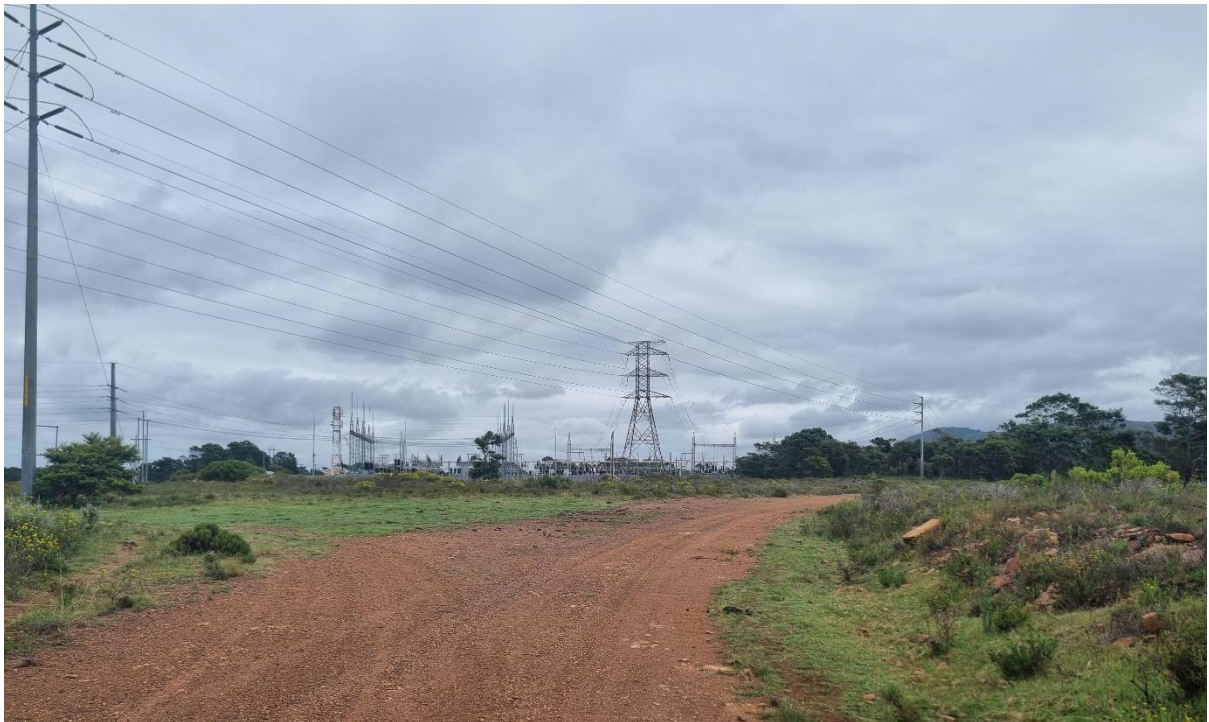
Figure 23: View of the existing Eskom substation and associated transmission lines adjacent to the site
