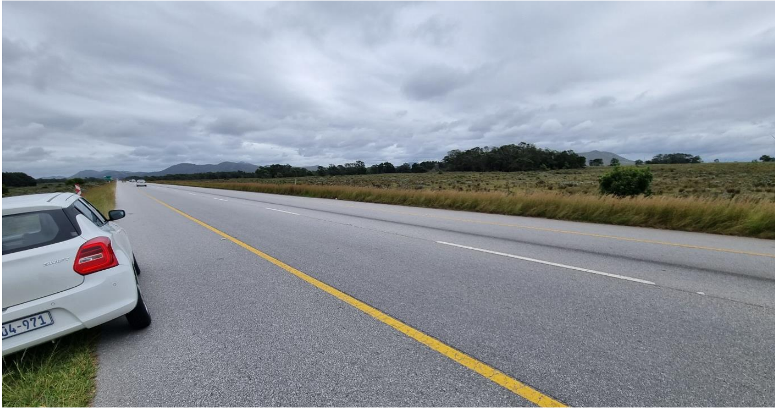
Figure 30: KOP 1_View towards the site from the N2 looking west, showing a dense group of trees in the background that screens views towards the site
