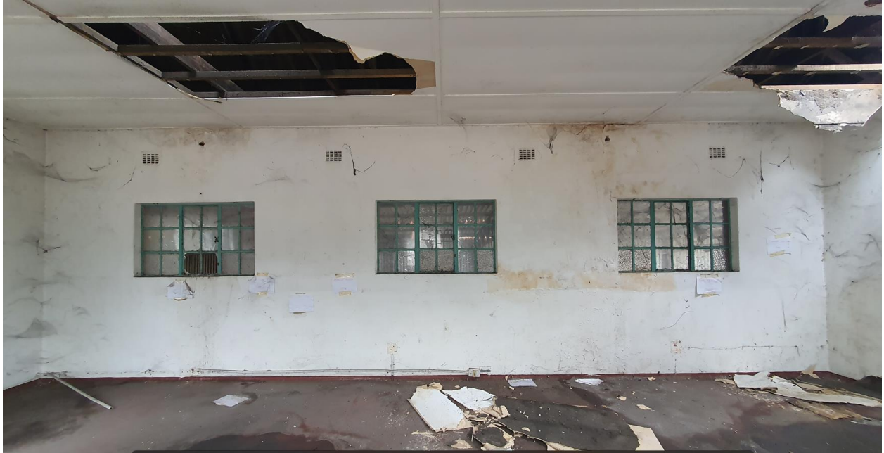
First Floor view
