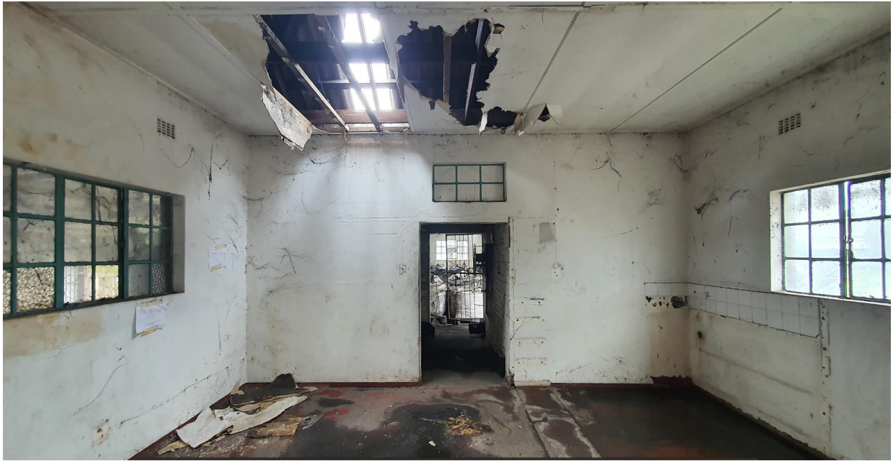
First Floor View
