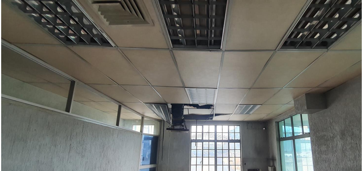
Typical Ceiling Finish
