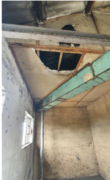
Thrid Floor Grain penetration through roof and floor
