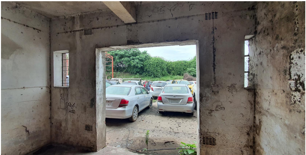
Building C Entrance Internal View
