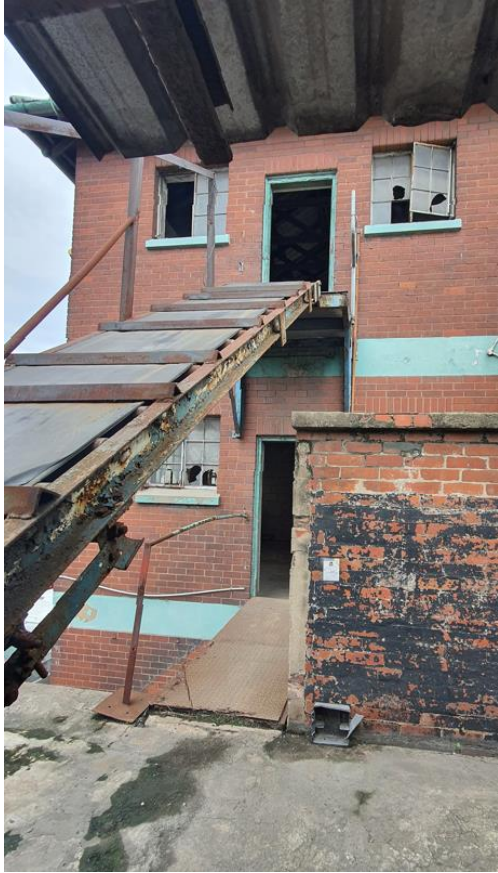
Entrance to building B from Building C
