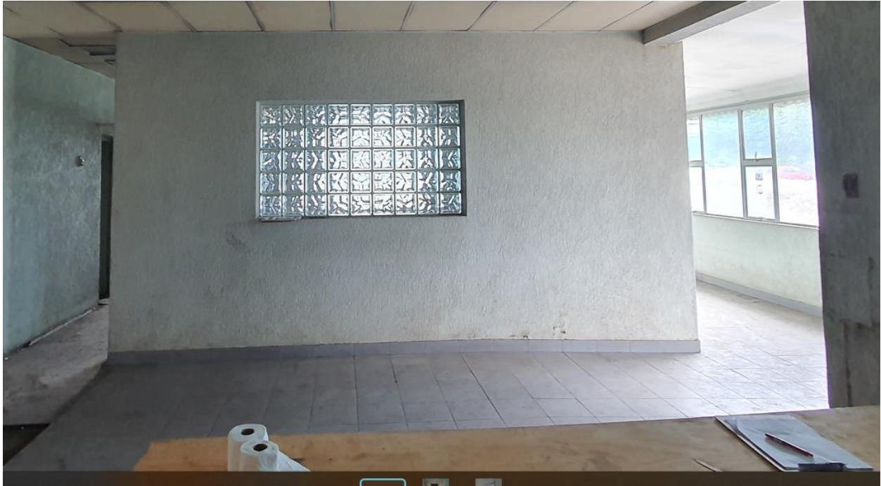
Typical internal wall finishes.
