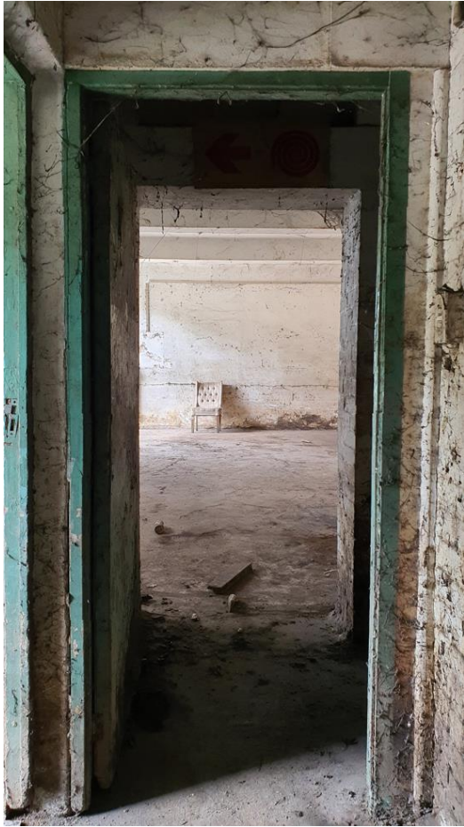
Ground Floor Passage
