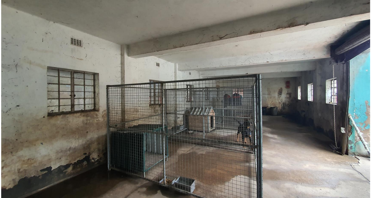
Ground Floor Workshop Area
