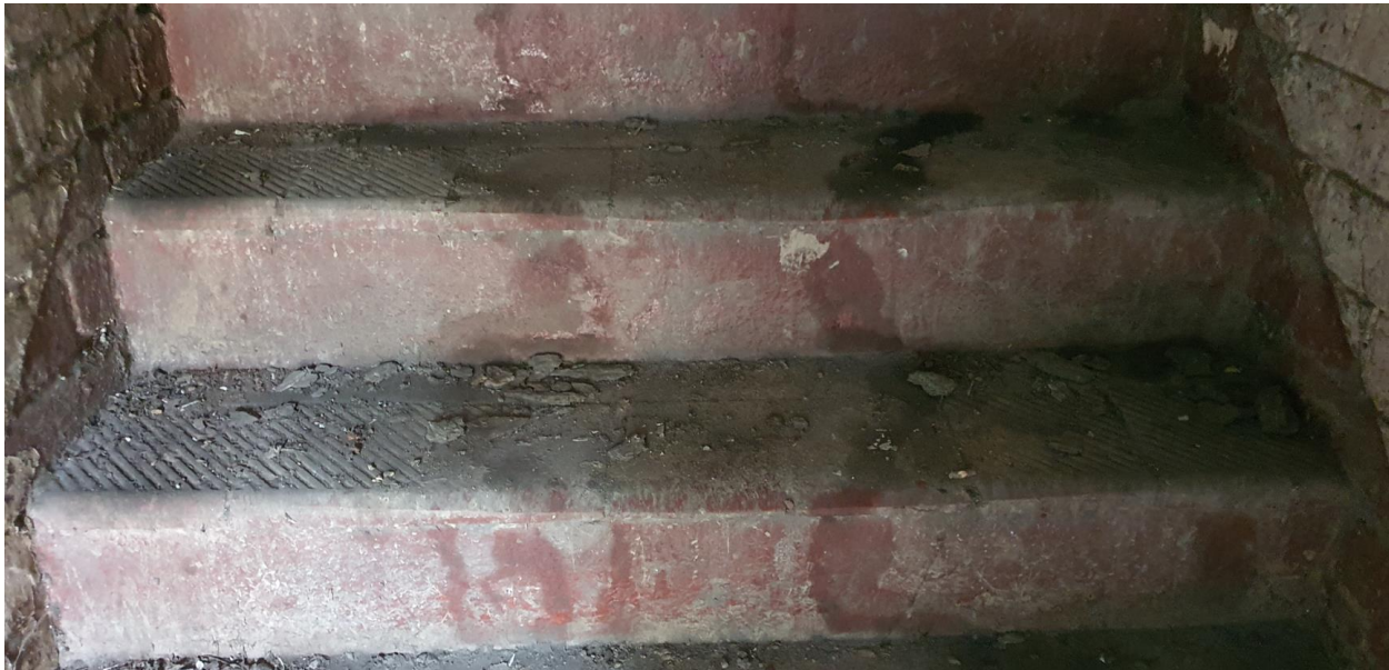
Stair Treads to First Floor
