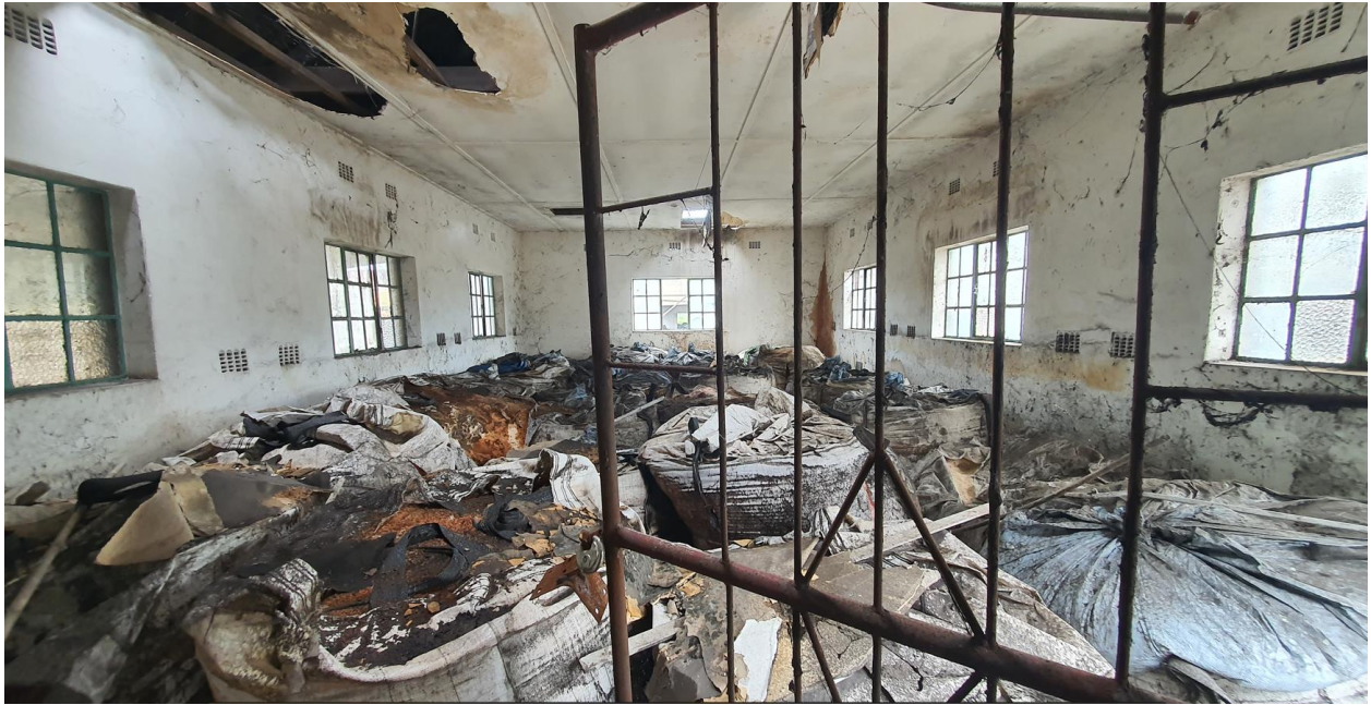
First Floor View
