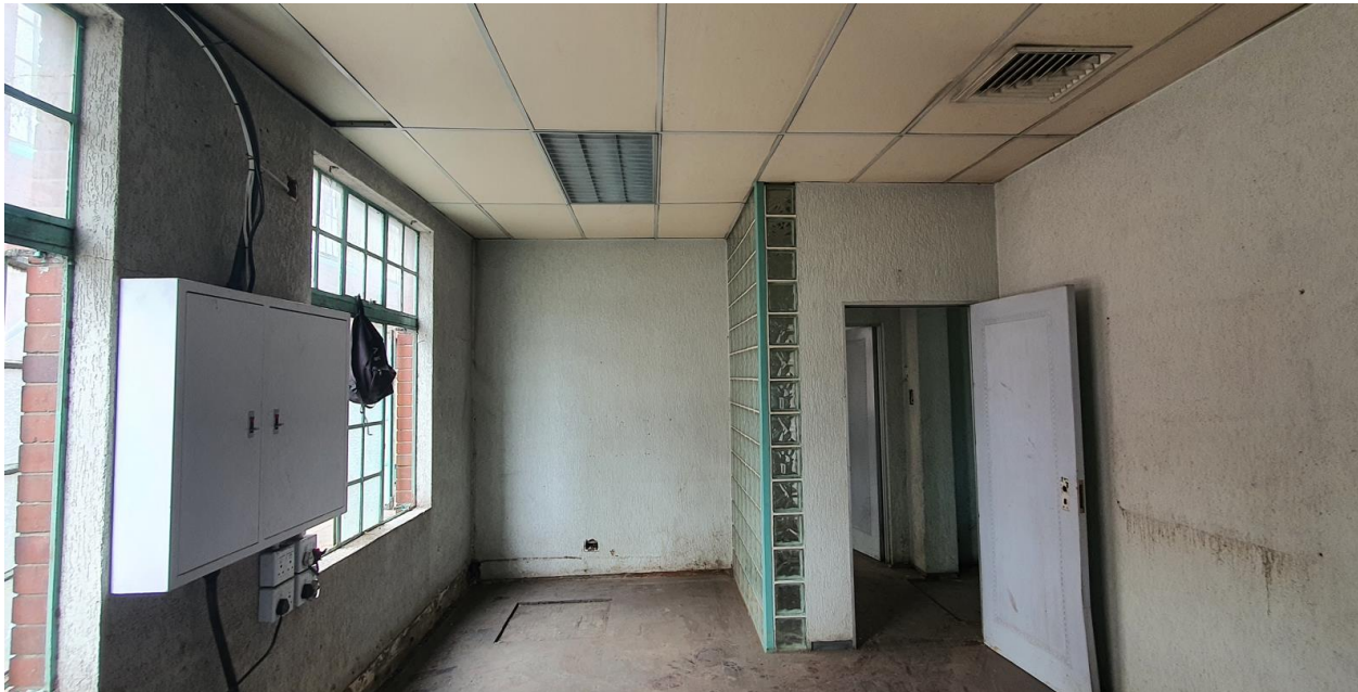
Typical Wall finishes in Building A. Note the modern glass blocks being used as well as the absence of timber skirtings. All doors were damaged during the floods. For more pictures, please see attached folder.
