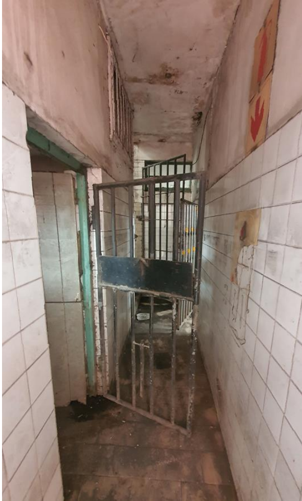
Building C Ground Floor Passage
