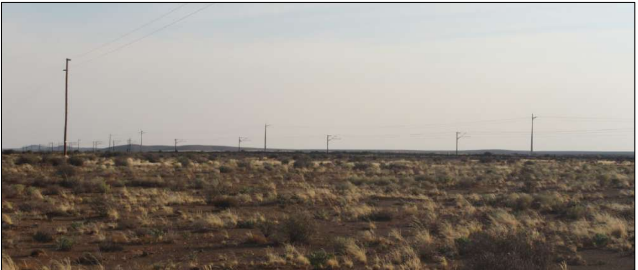
Figure 6: View towards the southwest towards the point where the Kokerboom 1 section of the powerline would cross the railway line.
