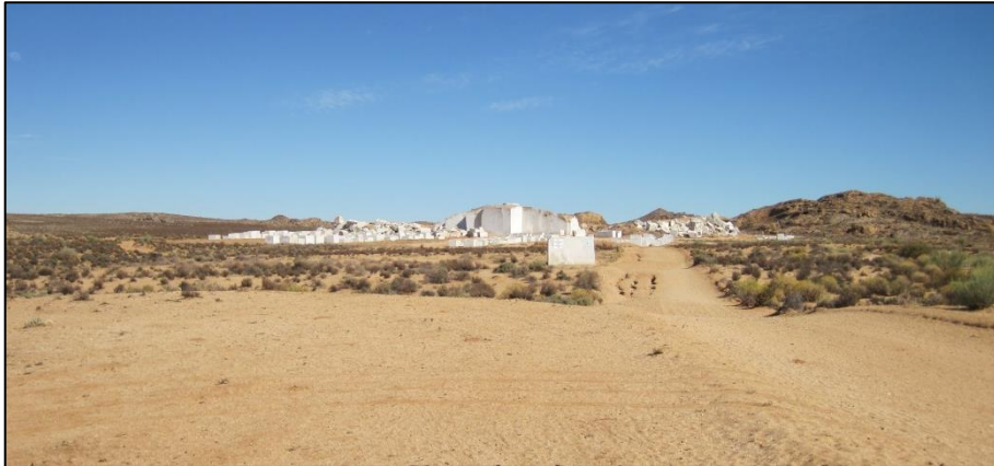
Plate 22: View of Rondeberg quarry looking north.
