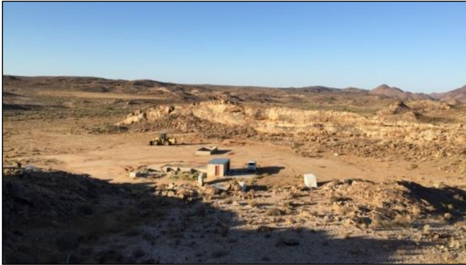
Plate 6: Looking north over the existing infrastructure
