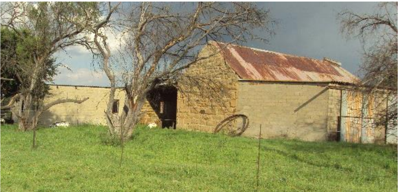
Figure 27: Rear view of the sandstone barn/shed, showing later additions
