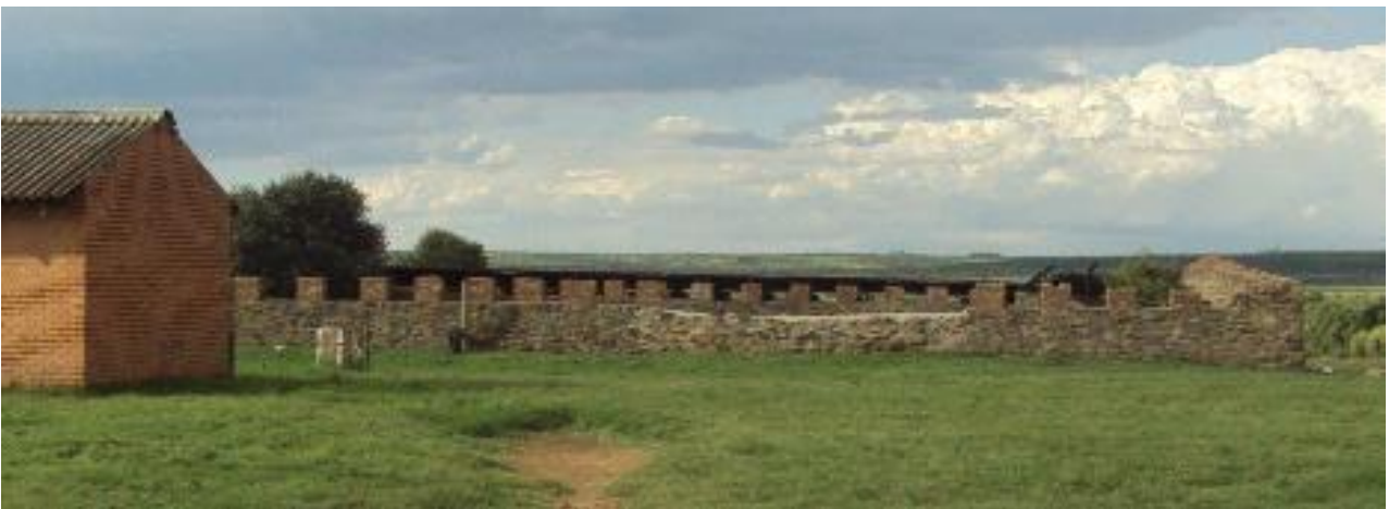
Figure 29: View of the historical kraal, showing brick additions to the stonework
