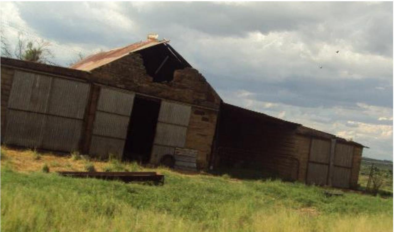
Figure 26: View of historical bar/shed structure, showing later additions
