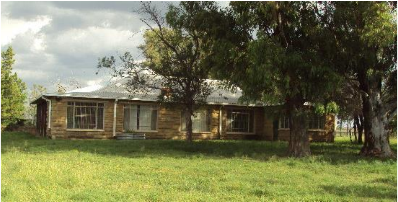
Figure 24: View of the western elevation of the sandstone farmhouse, facing the gravel road
