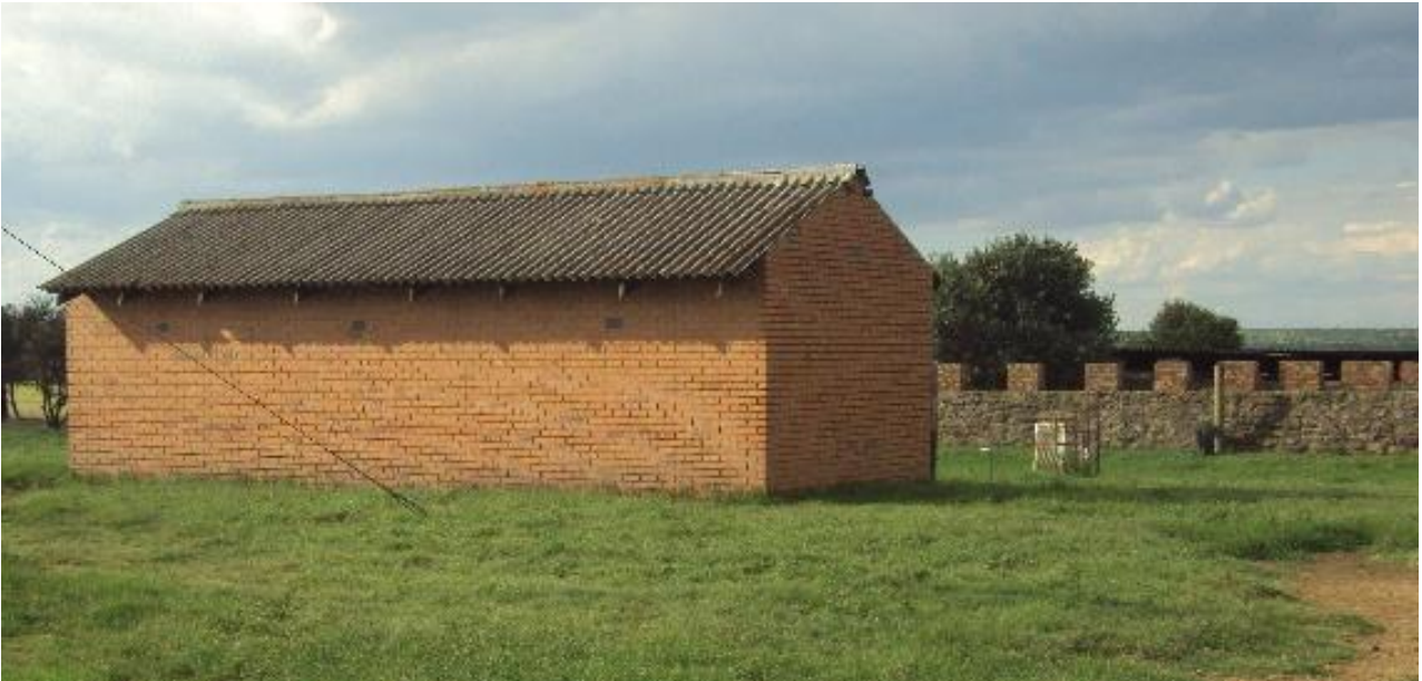
Figure 28: View of the more recent barn/shed, showing part of the historical stone kraal
