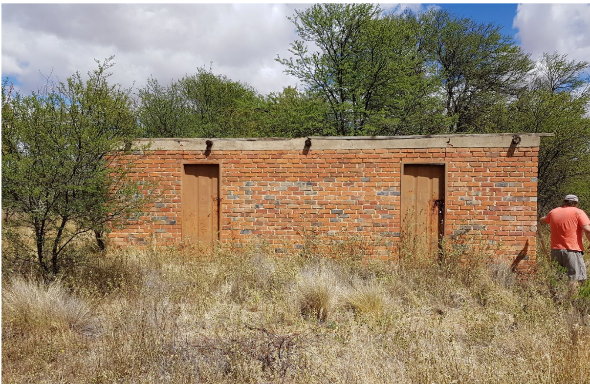
Figure 18: Front view of building
