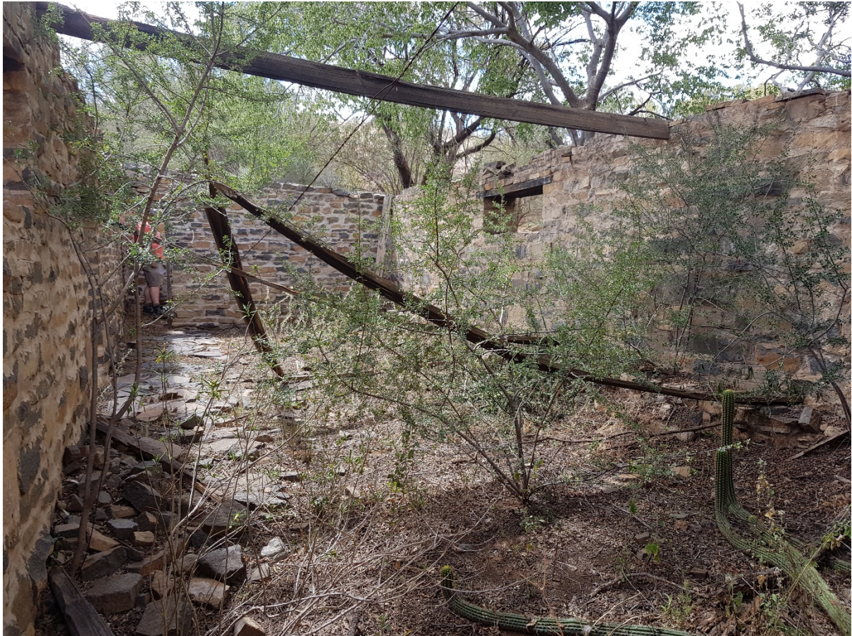
Figure 15: Interior view photographed from the side entrance with small room entrance at the far end. One in situ rafter. The interior connecting door space is considerably narrower at 77 cm as opposed to the two exterior entrances and is most likely designed to keep the mature animals out of that space.
