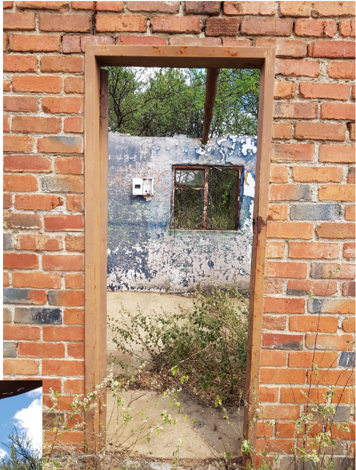
Figure 11: This building had an electricity supply and the walls show several successive layers of painting. The windows are of an average size, still commercially available.
