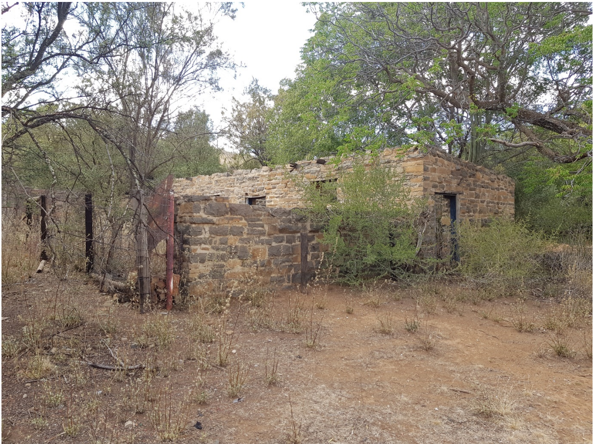
Figure 8: View from the north-western corner
