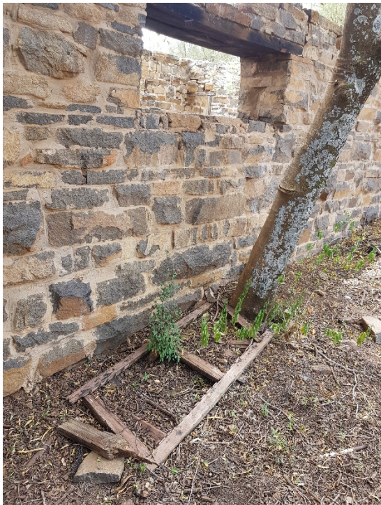
Figure 10: Wooden frame below window of rear wall
