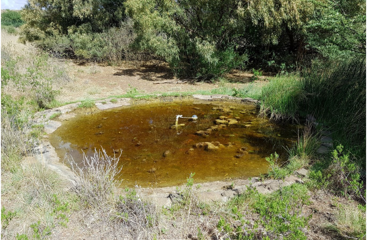
Figure 6: Cement lined shallow dam with Doppler pump
