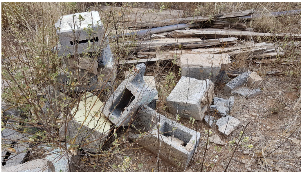
Figure 16: Building rubble from a demolished structure built with pre-cast cement bricks. The remaining foundation indicate it to be a two-roomed structure, two adjacent 3.5 X 3.5 m rooms, each with their own entrance.
