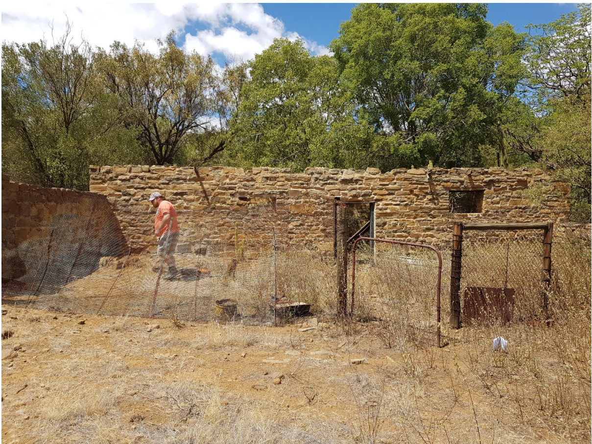
Figure 12: Front view (northern side) of barn showing wire fence and gate
