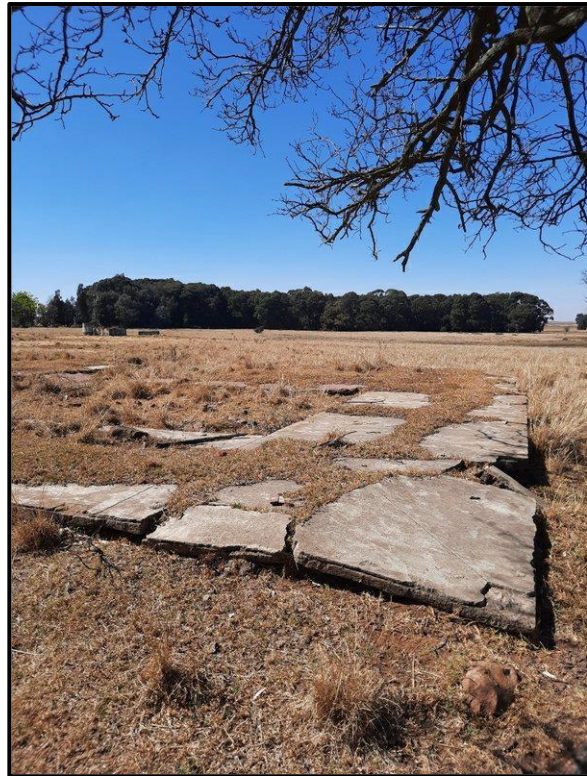
Figure 8.11. Foundations at Waypoint 104.
