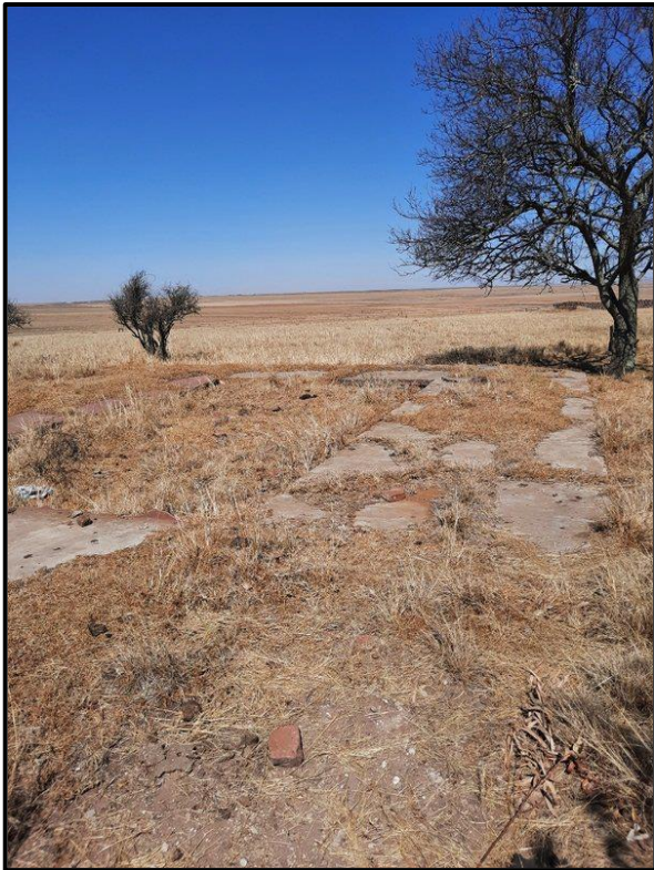
Figure 8.10. Foundations at Waypoint 104.
