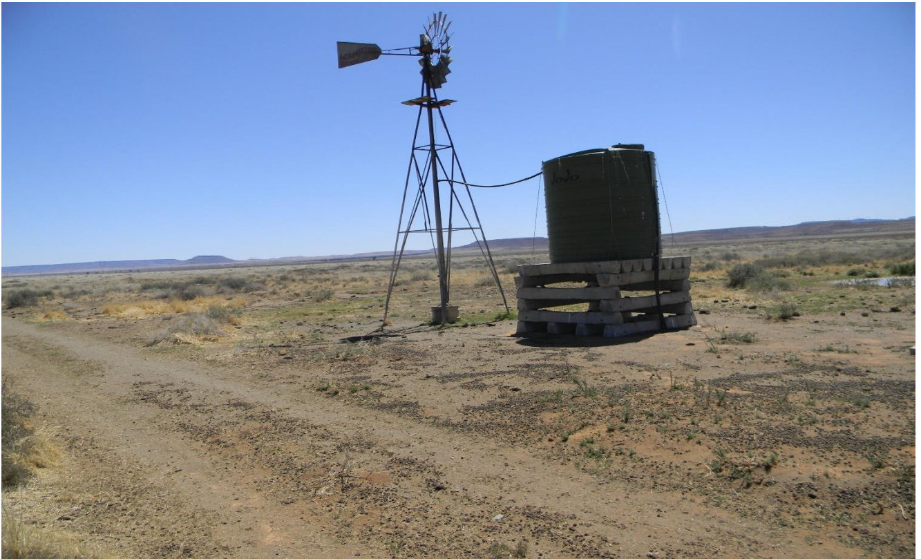
Plate 21: showing one of the several wind mills within the proposed development site.
