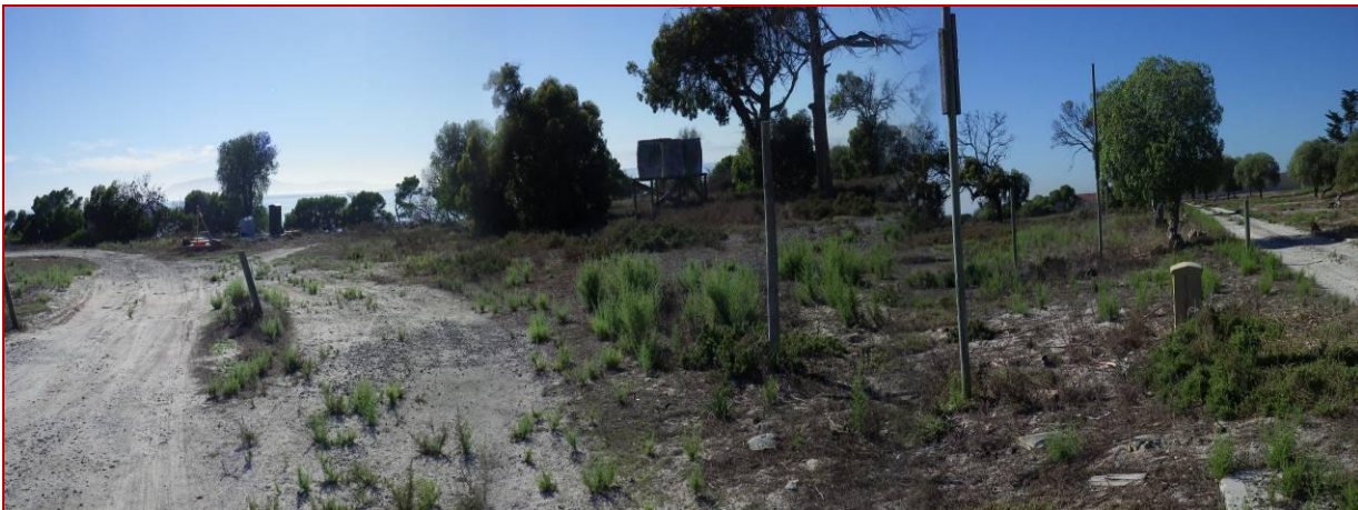
Fig. 9 Panorama of the site under investigation, facing east: to the left – in the back - the three concrete sewage pump stations, center: 3 fresh water tanks on a platform, to the right an electrical distribution box, wooden poles. Note the primary gravel roads and paths.
