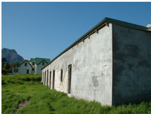
Stables in central part of the property
