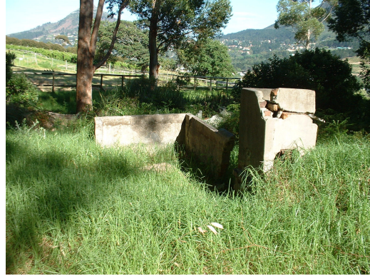
Derelict masonry water intake
