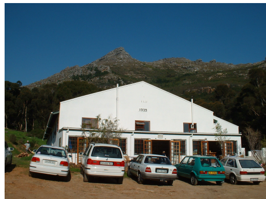
Front of old dairy with gable dated 1939
