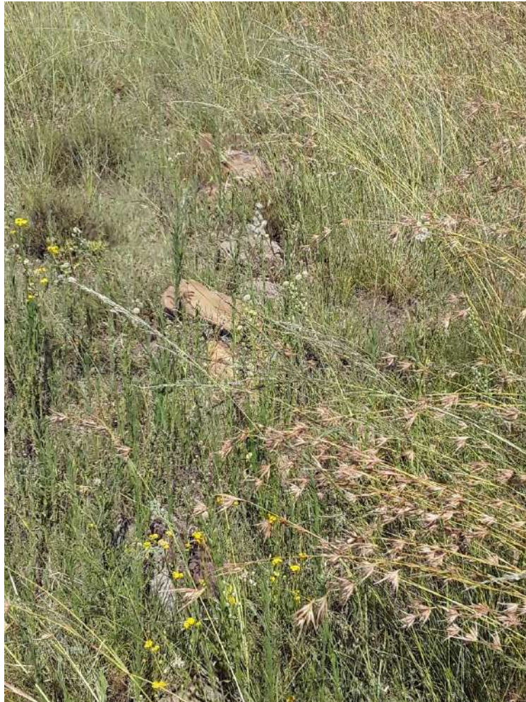
Figure 21: View of a line of stones forming the foundation wall of a structure
