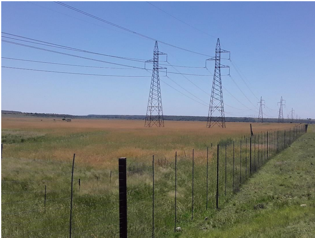
Figure 7: View of powerline running adjacent to the western boundary of the project footprint (Alternative 1)
