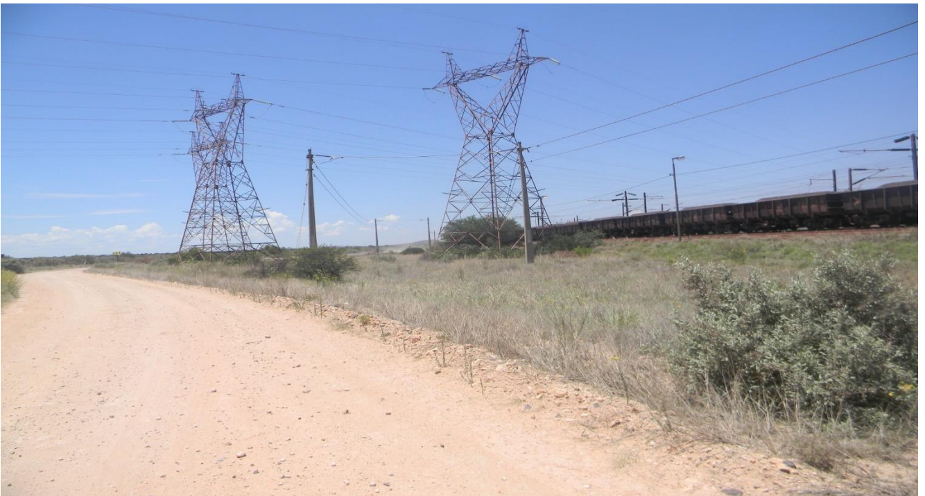
Plate 8: showing structures dotted within the proposed development site.
