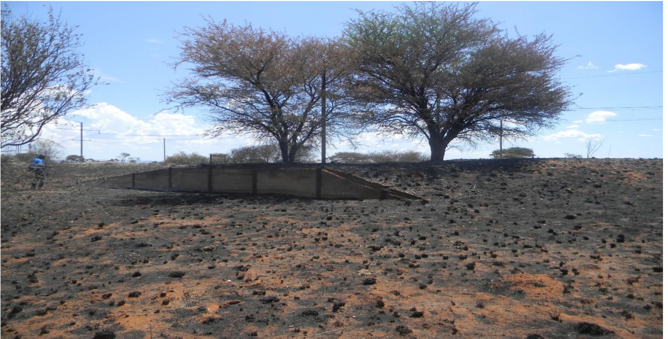
Plate 21: showing degraded sections of the proposed site.
