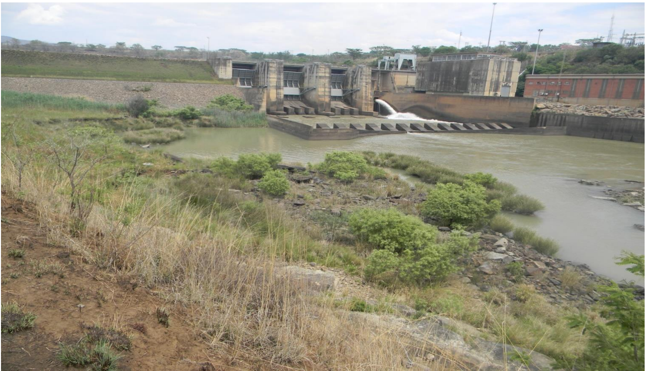
Plate 7: showing riverbanks to be rehabilitated and the dam structures.
