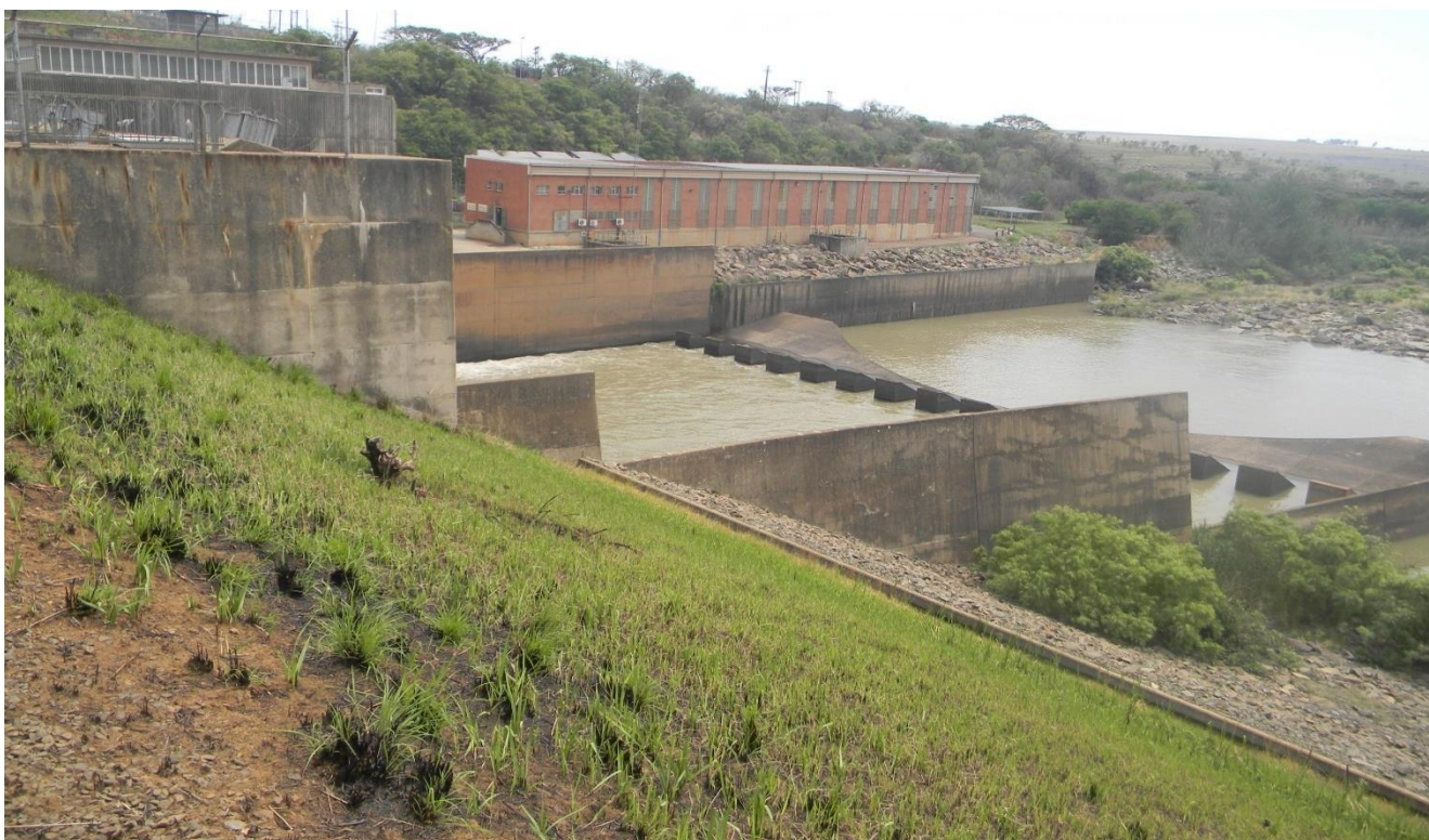
Plate 5: Showing Driel Barrage Water works treatment plant.
