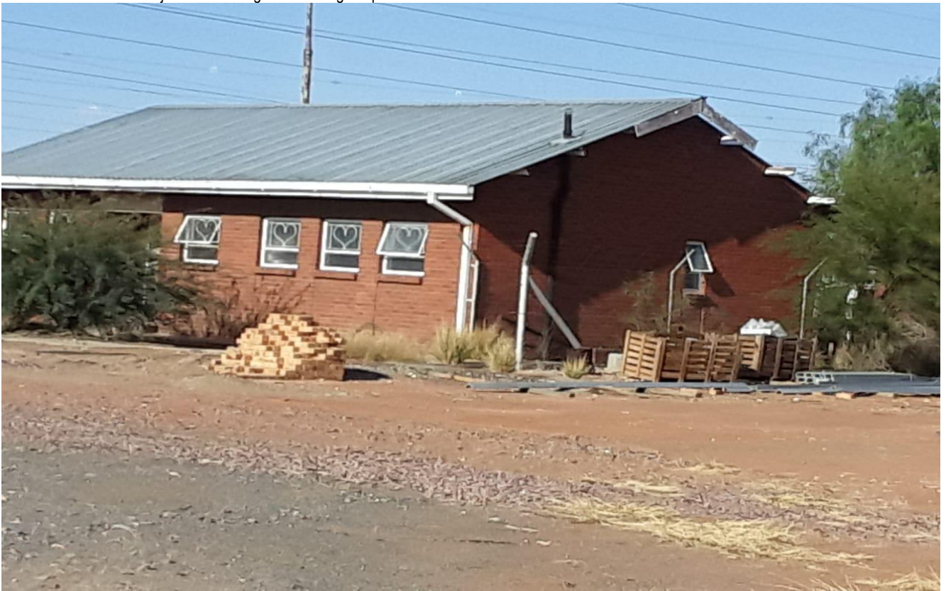
Plate 11: Photo 11: View of buildings at the Cuprum Substation (Photograph © by Author 2021).
