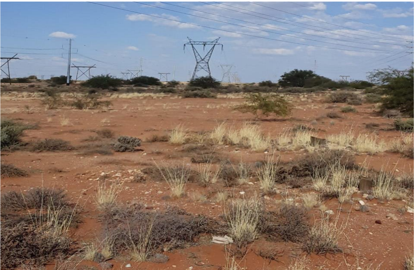
Plate 10: Photo 10: View of existing powerlines connecting to the substation earmarked for extension (Photograph © by Author 2021).
