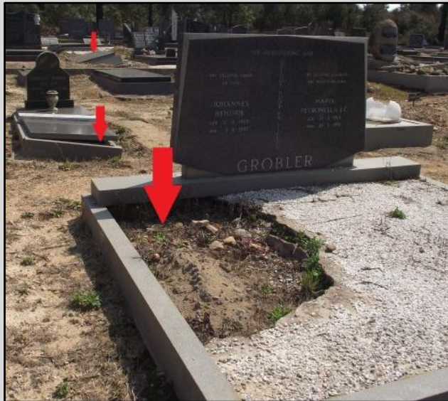
Figure 94 – Extent of visible subsidence
