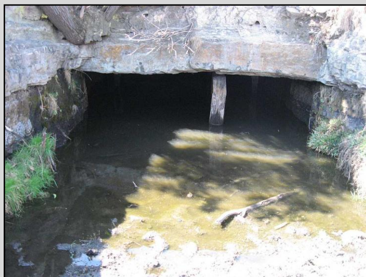
Figure 39 – PP 013: Close-up of shaft entrance
