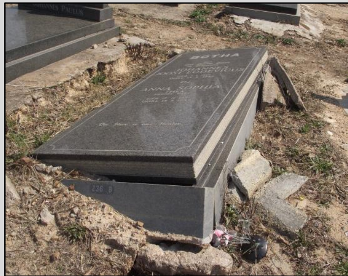
Figure 95 – Damaged and subsiding grave slab
