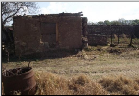
Figure 19 – PP 006: Close-up of dwelling addition
