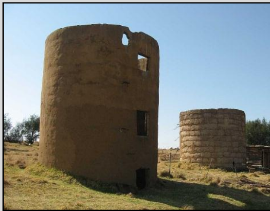
Figure 33 – PP011: Two silos
