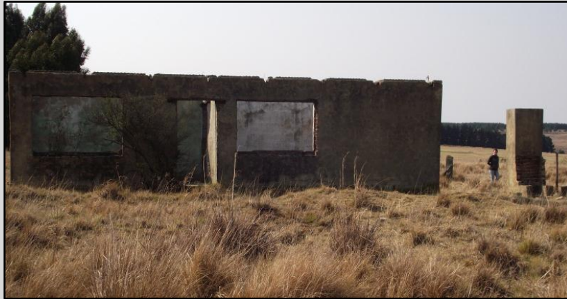
Figure 60 – PP 025: Ruins of farmworker dwelling and “donkey” structure
