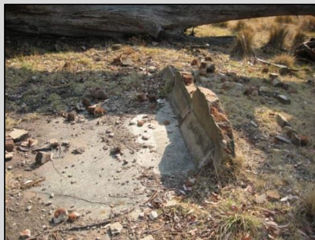
Figure 62 – PP 025: Close-up of shed wall
