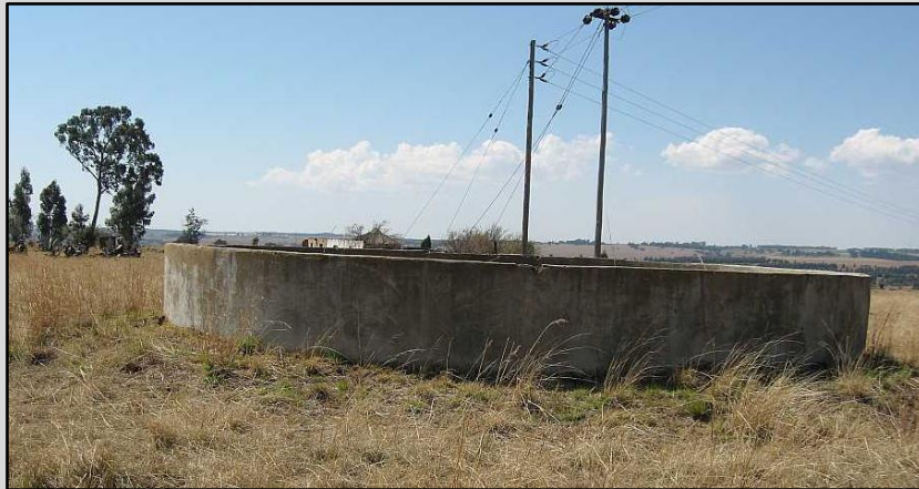
Figure 51 - PP 020: Cement Dam
