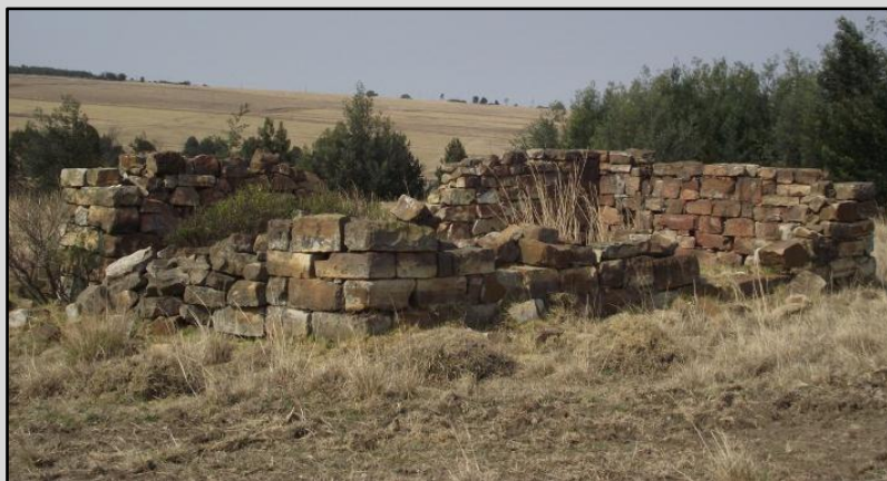
Figure 65 – PP 027: Ruins of sandstone shed
