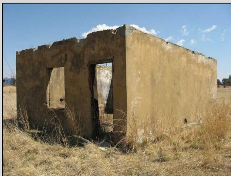
Figure 52 – PP 020: Brick structure
