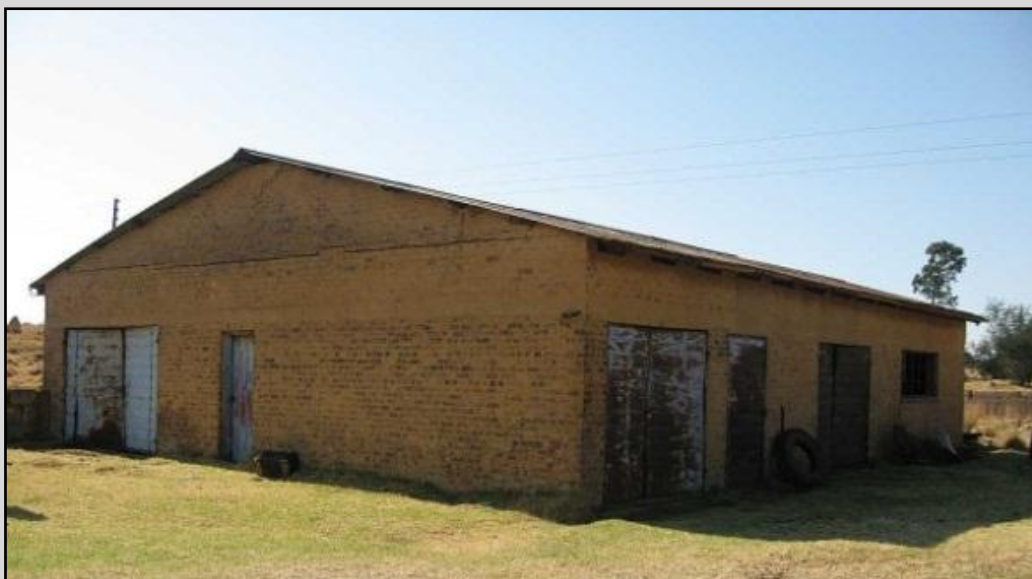
Figure 31 - PP011: Brick shed
