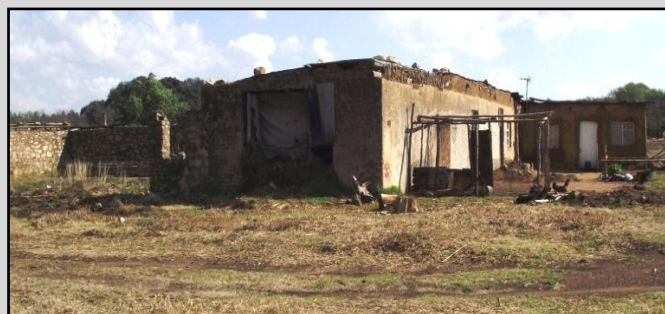
Figure 20 – PP 006: Close-up of dwelling addition
