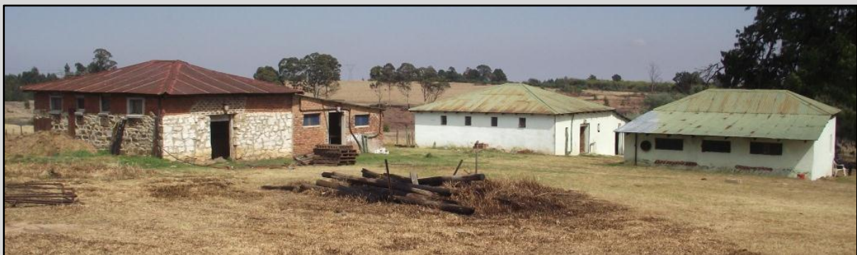
Figure 9 – PP001: Pigsty and two sheds/Storerooms
