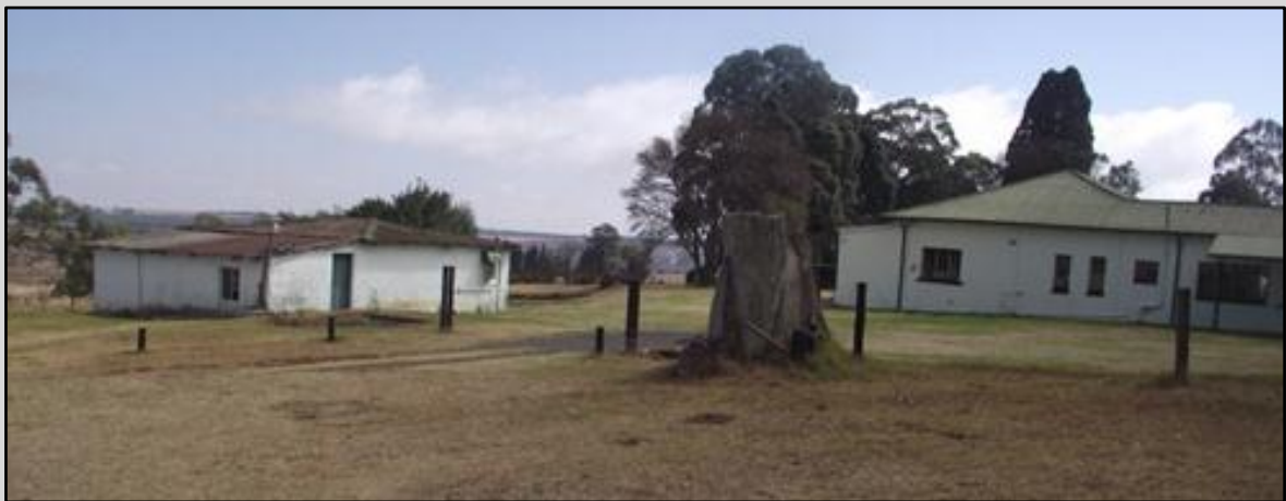
Figure 8 – PP 001: Main house and storeroom/shed
