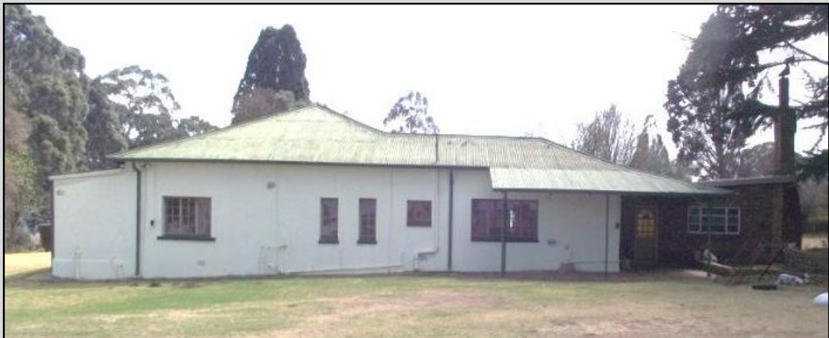
Figure 7 – PP 001: Main farmhouse building
