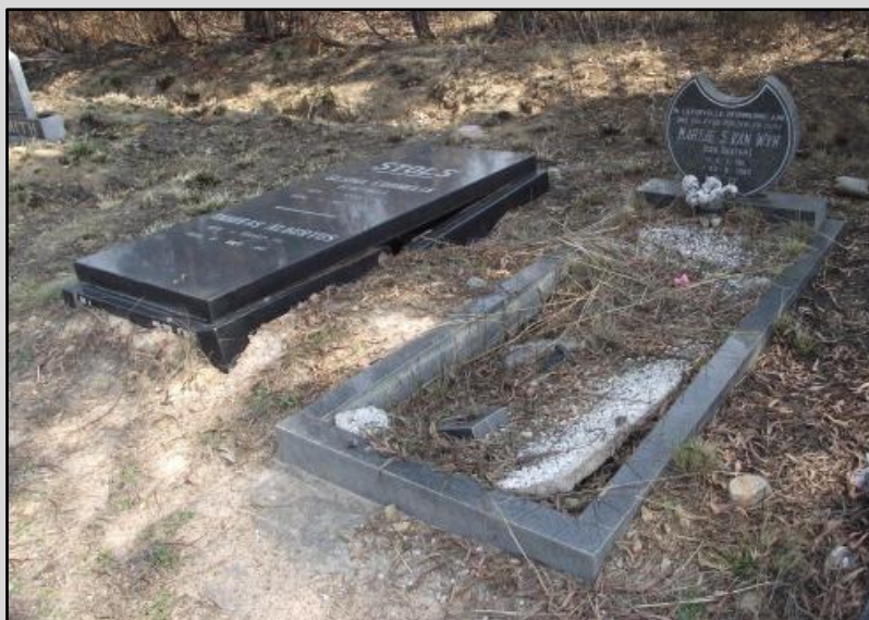
Figure 93 – Evidence of subsidence
