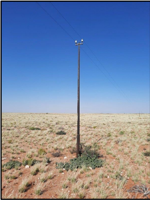
Figure 7.5. Cast iron telephone poles.
