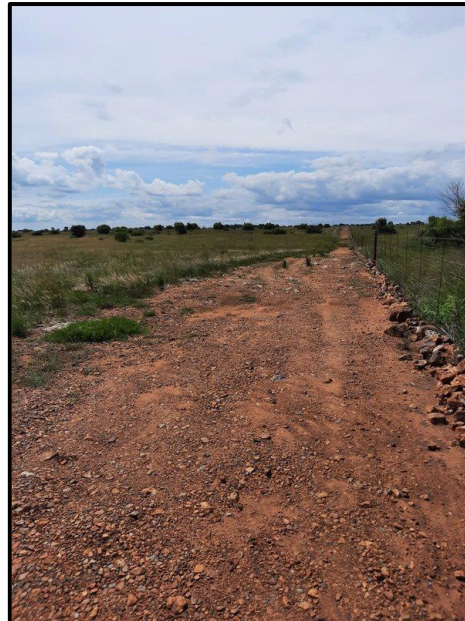
Figure 8.3. Exposed gravel layer in a freshly scraped road.
