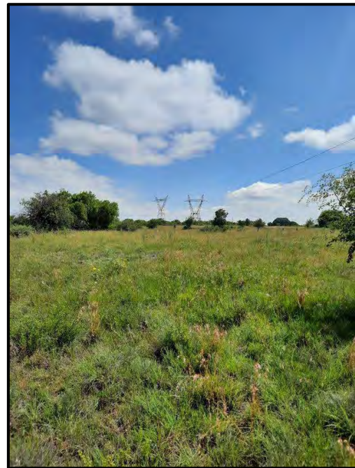
Figure 5.4. Powerline in the study area.
